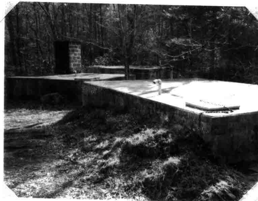
THREE RESERVOIRS WITH A COMBINED CAPACITY OF 51,000 GALLONS SERVING CADES COVE CAMPGROUND
