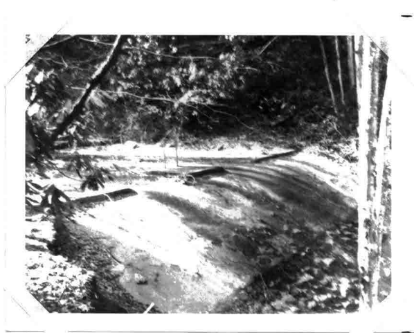
THIS DAM ON A TRIBUTARY STREAM FORMED THE ORIGINAL INTAKE STRUCTURE FOR THE SYSTEM
