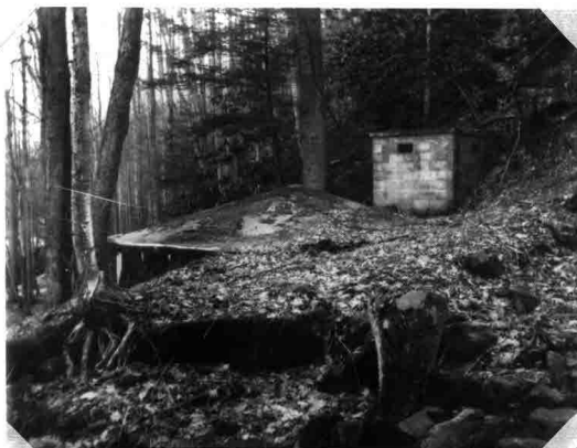
RESERVOIR AND CHLORINATOR HOUSE
