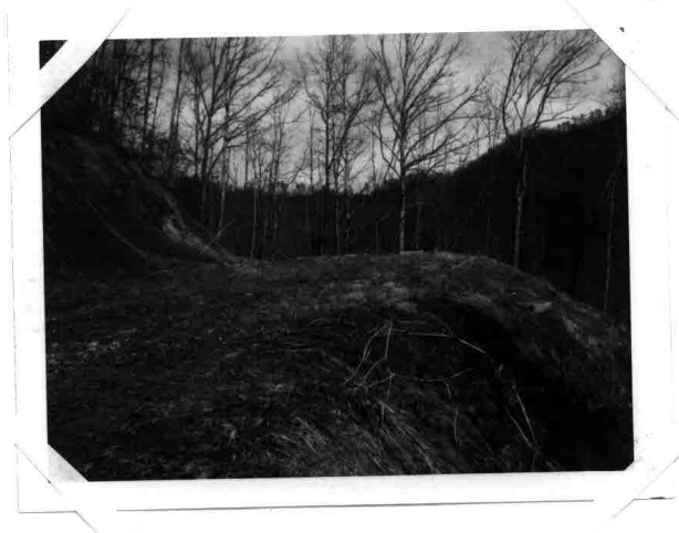
Right: A 20,000 Gallon Reinforced Concrete Reservoir Buried on a Hillside Serving Collins Creek Picnic Area
