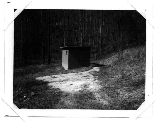
Left: Pump House at Collins Creek Containing a Deep Well Pump and Water Neutralizer
