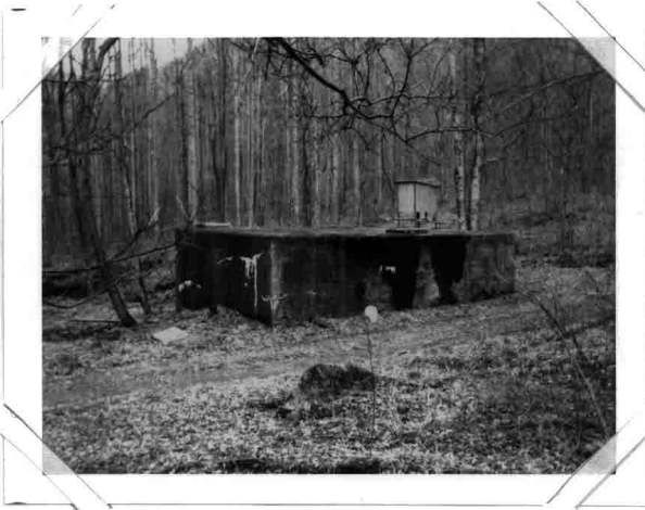
25,000 GALLON RESERVOIR WITH CHLORINATOR HOUSE
