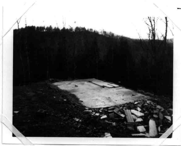
10,000 GALLON REINFORCED CONCRETE RESERVOIR BURIED ON HILLSIDE
