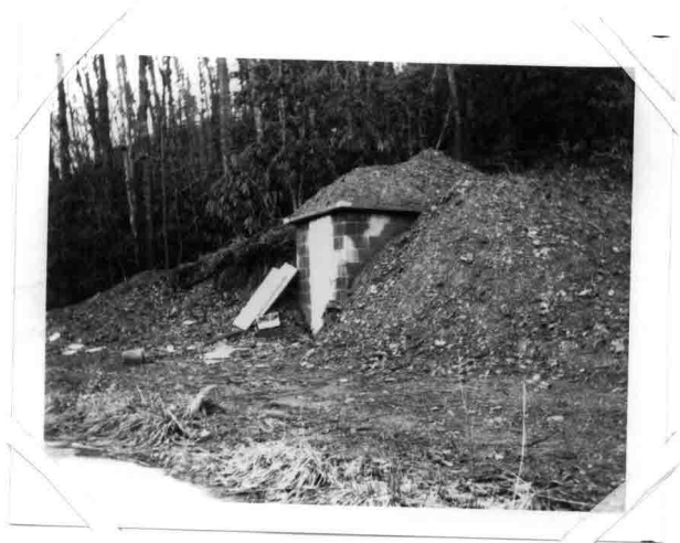
CHLORINATOR HOUSE ADJACENT TO RESERVOIR BURIED IN HILLSIDE
