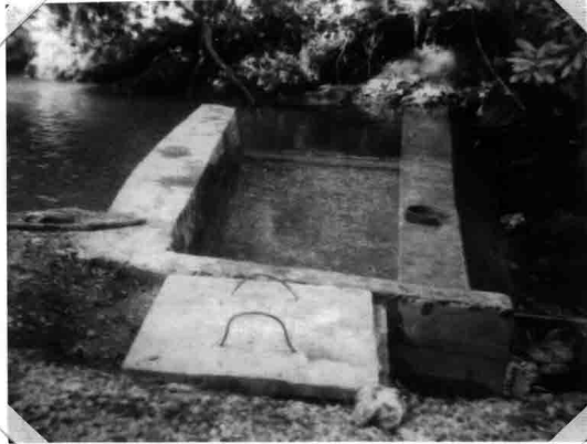
INTAKE STRUCTURE AT DEEP CREEK SHOWING THE SETTLING BASIN, WINGWALL, DAM, FILTER, AND COVERED COLLECTION BOX
