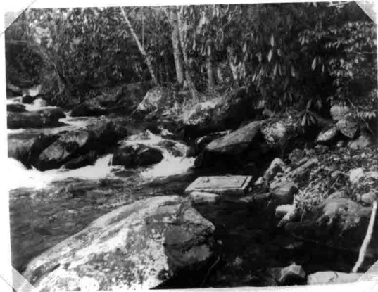
WATER INTAKE FOR ELKMONT CAMPGROUND LOCATED ON JAKES CREEK
