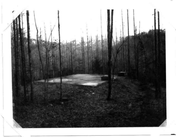
A 50,000 GALLON, TWO COMPARTMENT RESERVOIR AT ELKMONT CAMPGROUND
