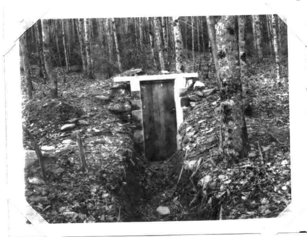
THE CHLORINATOR HOUSE AT THE RESERVOIR OF THE ELKMONT CAMPGROUND WATER SYSTEM
