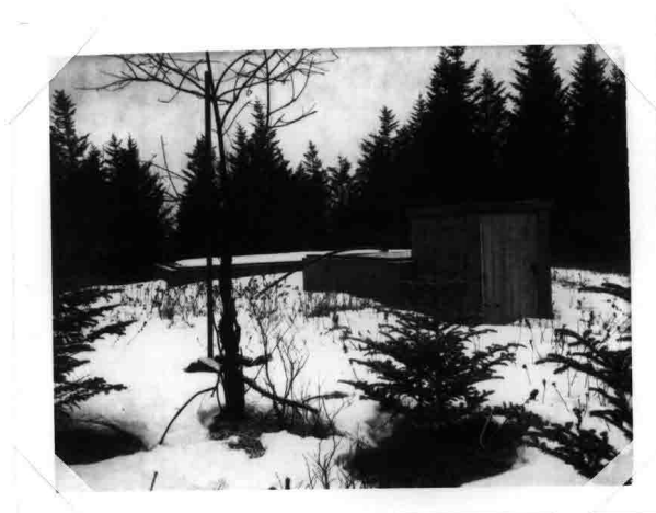
CHLORINATOR AND FILTER BED
