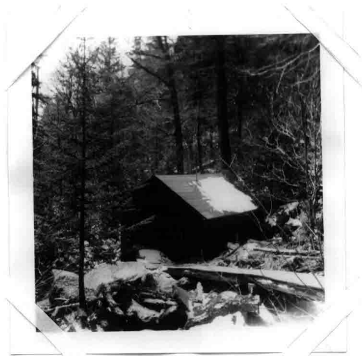
Pump House for the Forney Ridge Water System
