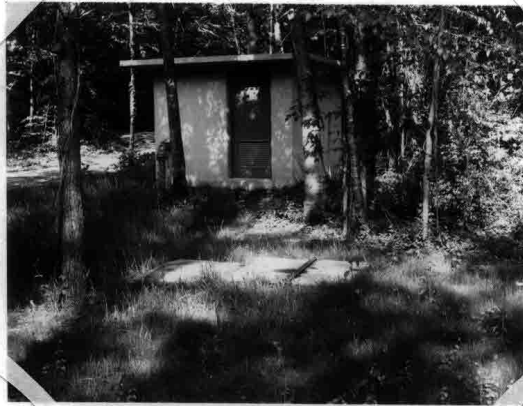
PUMP HOUSE AND METER BOX FOR HEADQUARTERS WATER SYSTEM
