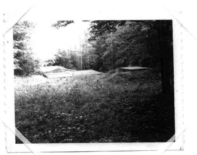
25,000 AND 50,000 GALLON RESERVOIRS AND SAND FILTER FOR HEADQUARTERS WATER SYSTEM
