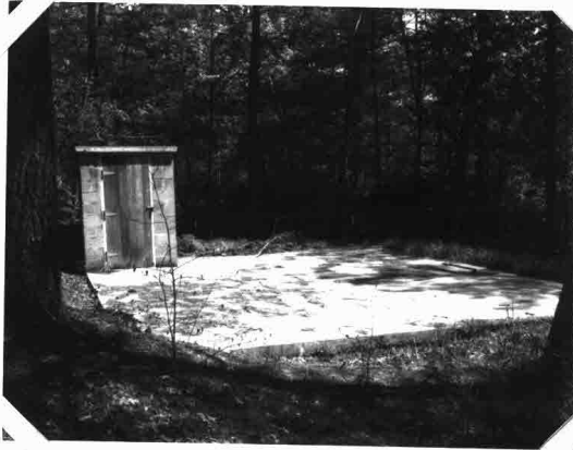
CHLORINATOR HOUSE ATOP A 25,000 GALLON RESERVOIR
