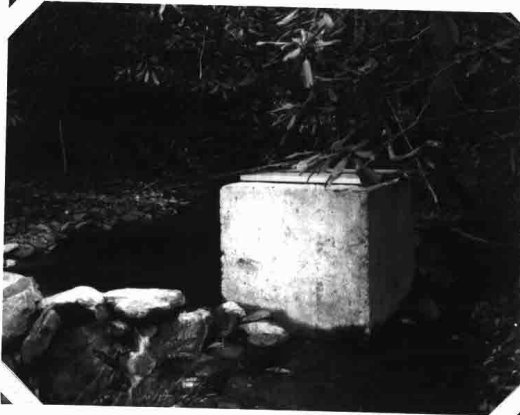
INTAKE STRUCTURE AT TRIBUTARY OF LITTLE GREENBRIER BRANCH
