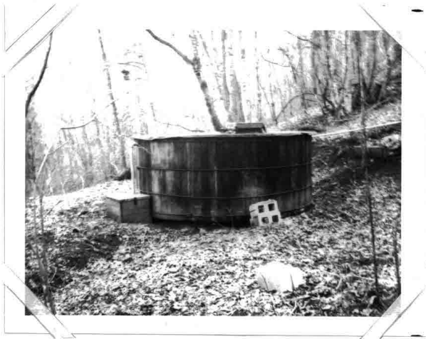
5,000 GALLON WOOD STAVE RESERVOIR
