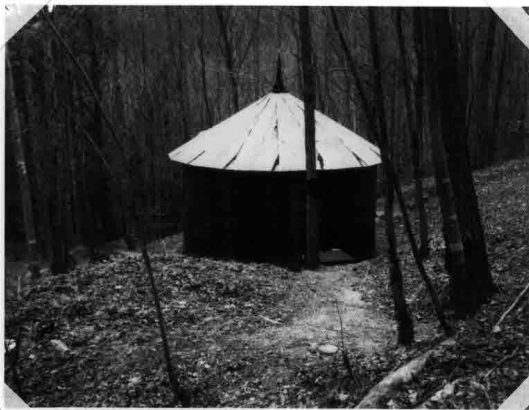
11,000 GALLON WOOD STAVE RESERVOIR
