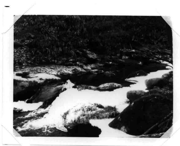
WATER INTAKE CONSISTING OF A ROCK DAM WITH A 2" DIAMETER SCREENED INLET BEHIND THE DAM
