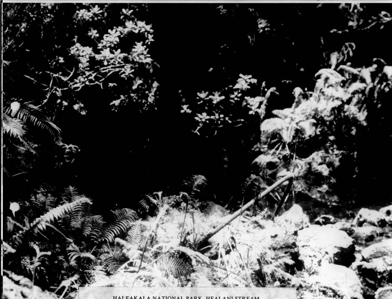
HALEAKALA NATIONAL PARK, HEALANI STREAM. Abandoned piping to former water supply pool for Kaupo Ranch. 06/11/93
