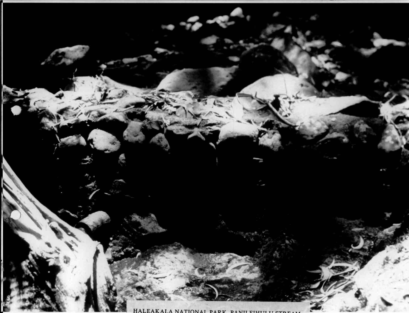
HALEAKALA NATIONAL PARK, PANILEIHULU STREAM Kaupō water supply intake dam. 6/11/93
