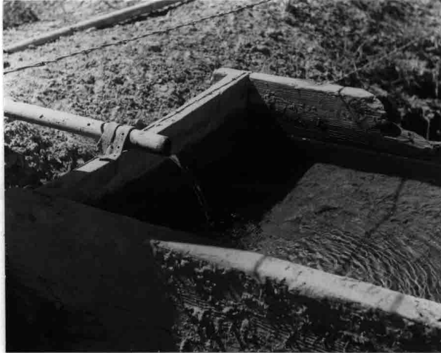
No. 5. Overflow from storage tank in No. 1 flows through this pipe and into trough for stock watering.
