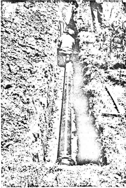
6" C.I. WATER MAIN UNDER CONSTRUCTION FROM WELL NO. 1 TO VISITOR-CONTACT STATION, BLDG. NO. 276 COLBERT PARK, SECTION 2-C NATCHEZ TRACE PARKWAY
