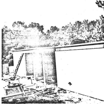
VISITOR-CONTACT STATION UNDER CONSTRUCTION, BLDG.NO. 276 COLBERT PARK, SECTION 2-C NATCHEZ TRACE PARKWAY
