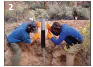
(1) Hiking to well installation site and (2) Installing a well, East Fork of the Virgin River, Zion NP.
