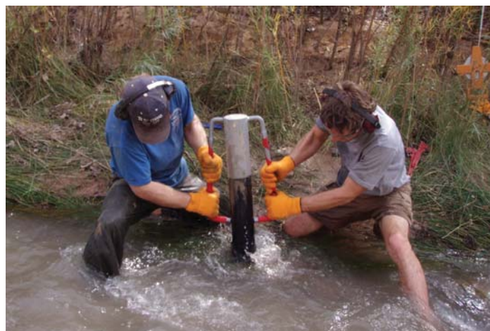
Installing a well on the East Fork of the Virgin River, Zion NP.
