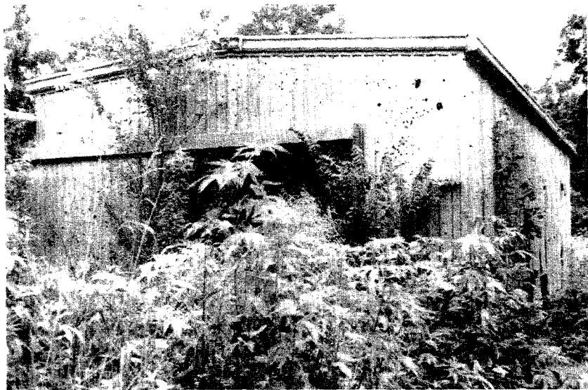
Photo 19. Illegal Pumphouse, Barataria District.
