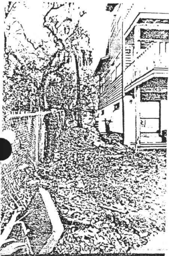
Tract 01-129 - Photographer facing south, ranger standing on boundary (note proximity of fence to residence)
