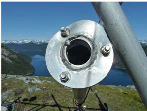
Figure 26. The 20 ft mast broke at the junction weld (McArthur Pass RAWS). Upper 10 ft section and both halves of the junction are visible.
