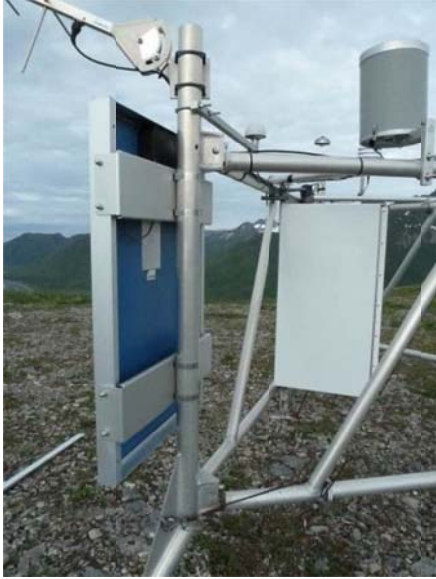
Figure 12. Both welds on the south (left) corner of the NW tri-leg tower panel section were broken (Fourpeaked RAWS).
