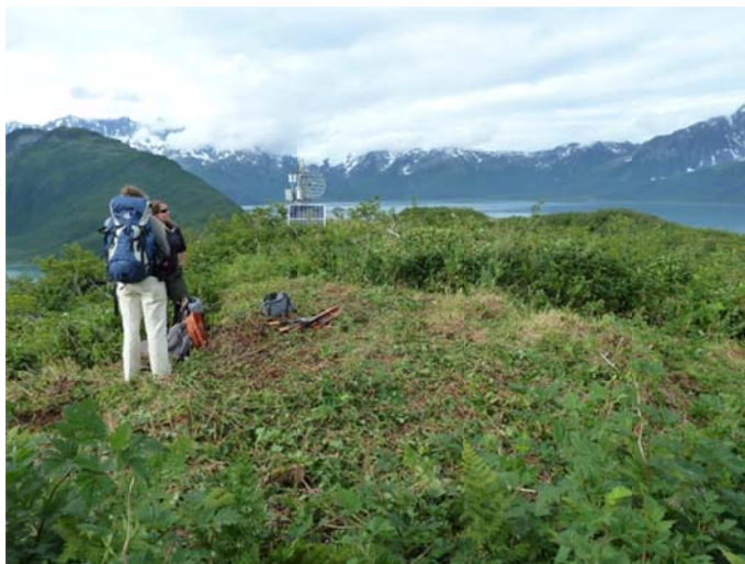
Figure 30. The weather station site after brushing alder and salmon berry (Pedersen Lagoon RAWS).
