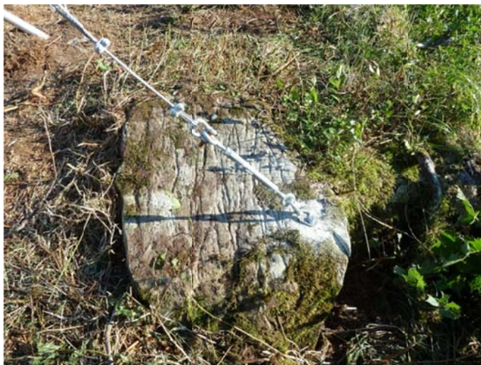
Figure 34. Guy line attached to an expansion bolt in bedrock (Pedersen Lagoon RAWS).
