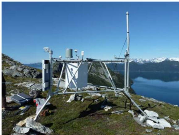
Figure 25. The wind sensors, 20 foot mast, and GOES antenna were wrecked (McArthur Pass RAWS).
