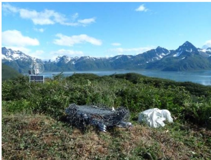
Figure 32. Sling net containing weather station (partially unpacked) and super sack with 500 lbs of beach rock (Pedersen Lagoon RAWS). The Alaska Sea Life Center's remote camera telemetry site is visible in the background of the picture.
