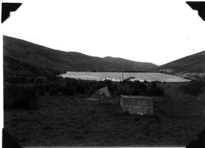
WR # 11 - Nunes Diversion Earthen dam and storage reservoir July 8, 1975
