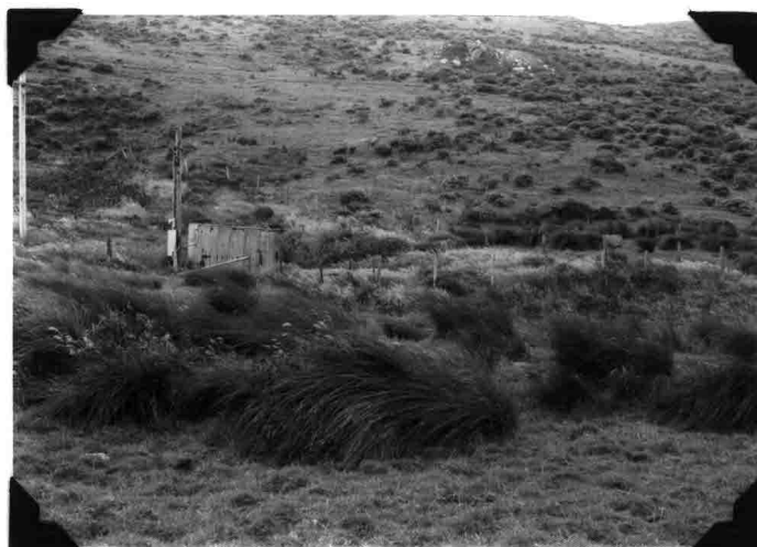
WR # 11 - Nunes Diversion Pumphouse and springbox (barely visible to the immediate right of the pumphouse) July 8, 1975
