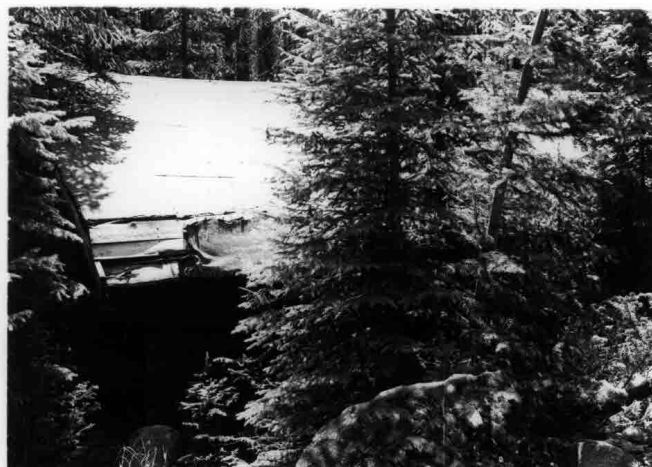
Grand Lake Lodge Powerhouse
