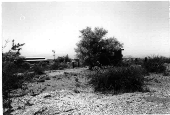
Looking Southwest, Headquarters Well #2 (known as Baker Well #3 by park personnel) is located in the pumphouse that is partially hidden by Palo Verde (in bloom). This site is in the extreme southwest corner of this Park Service property that is not within the park's boundaries.
