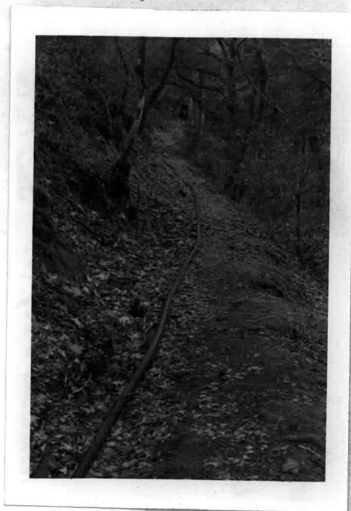
WHIS WR # 1 - South Liberty Gulch. Looking West, showing plastic pipeline from upper diversion dam. Water flows by gravity feed to a concrete storage tank for fire protection and seasonal irrigation (lawn and garden) use at NPS residences # 86 & 78.
