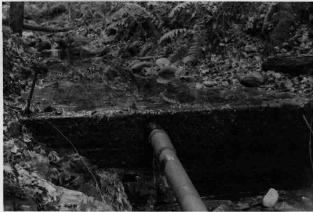
WHIS WR # 1 - South Liberty Gulch. Showing upper diversion dam and pipeline presently in use by NPS. Looking upstream, east. Werrell Jan 14, 1976
