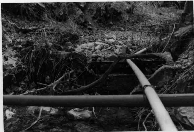
WHIS WR # 1 - South Liberty Gulch. Looking upstream, showing lower (unused) diversion dam. Werrell Jan 14, 1976
