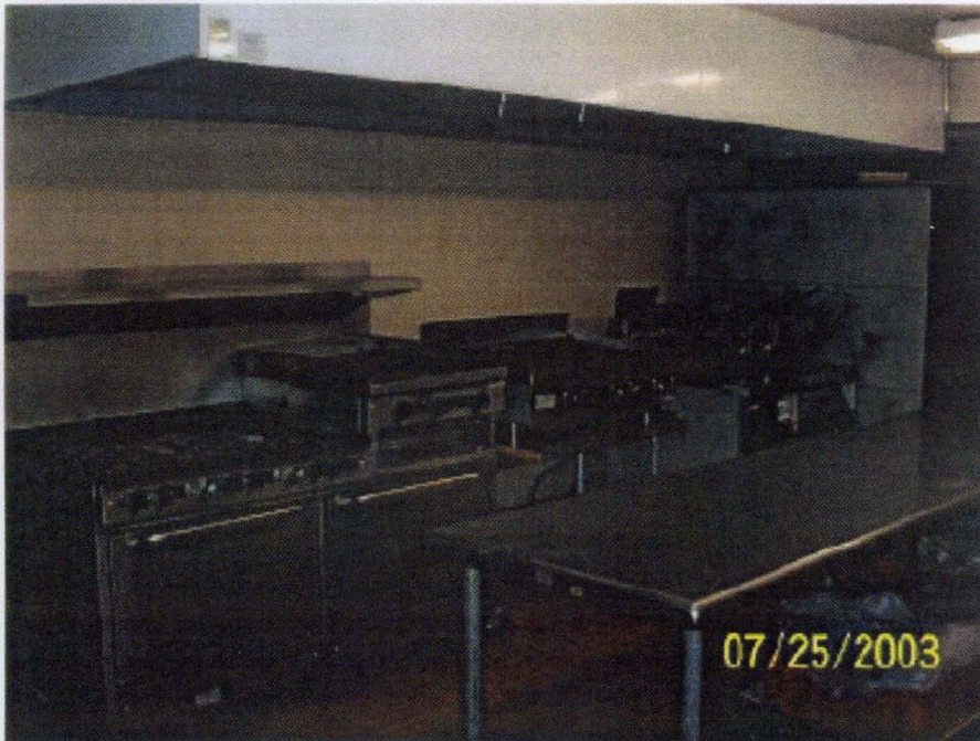
One of two kitchen facilities located at the Schoodic Education and Research Center.
