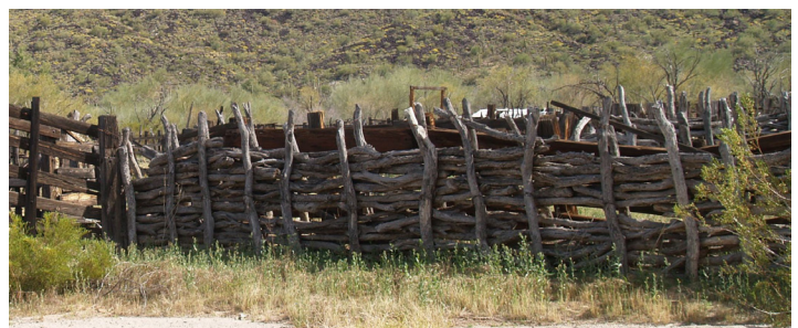
Figure 22: Constructed of interlocked, stacked mesquite rails supported by paired mesquite posts, this fencing represents a type made entirely of indigenous materials. The buried portions of the mesquite posts are highly susceptible to insect infestation and rot and as a result, many of the posts have failed allowing sections of this type of fence to collapse. Photo: Randall Skeirik, NPS
