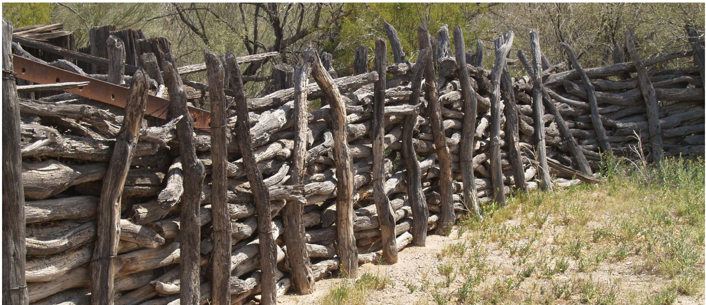
Figure 19: Constructed of interlocked, stacked mesquite poles supported by paired mesquite posts, this fencing represents a type made entirely of indigenous materials. The buried portions of the mesquite posts are highly susceptible to insect infestation and rot and as a result, many of the posts have failed allowing sections of this type of fence to collapse.
