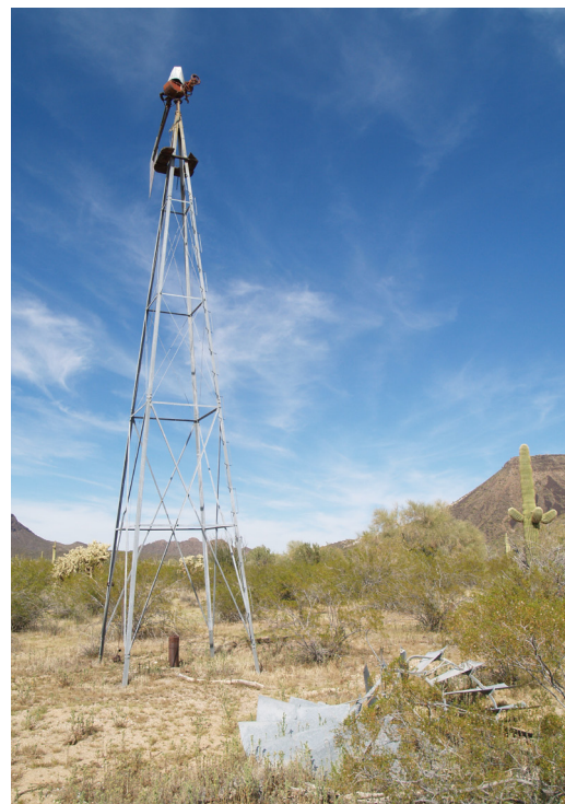
Figure 30: Windmill Number 3. Note the blades on the ground in the lower right. Photo: Randall Skeirik, NPS
