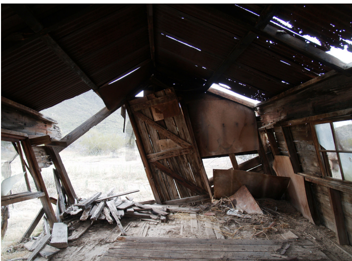
Figure 2: Interior view of Chico's House before and after the building was straightened and a temporary brace installed. This straightening was accomplished without tools, and braced with materials found on-site. Without permanent bracing, this building will soon collapse.
