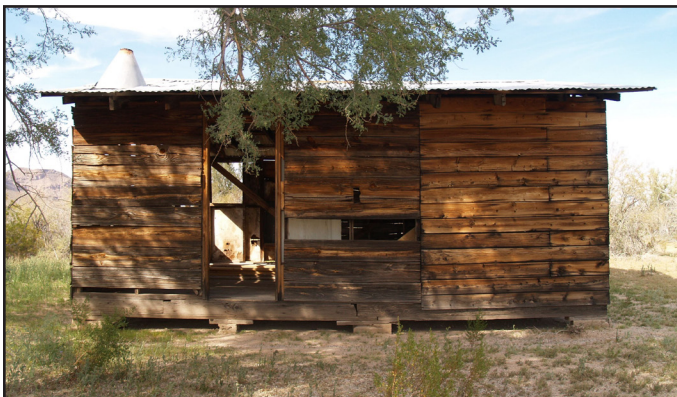
Figure 11: The Hay Barn. The vertical seam visible in the siding to the right of the door indicates where two different framing panels were joined. Because construction and siding types differ between some of the panels it can be inferred that this building was assembled with pieces removed from more than one structure. It is likely that the panels came from buildings originally associated with the nearby Growler Mine.
