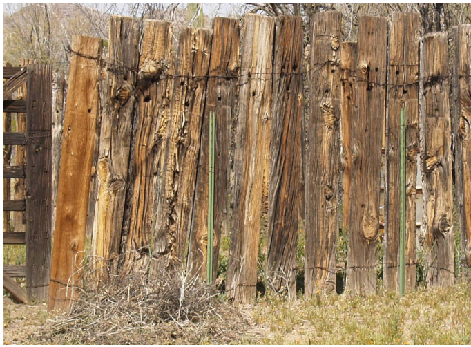
Figure 20: Stockade type fencing made from reused railroad ties. Even though these timbers were originally treated with creosote, the below-grade sections have deteriorated over the years. Note the green “T” posts that have been installed to help keep the fence upright. Photo: Randall Skeirik, NPS
