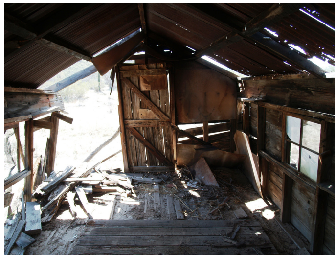
Figure 2: Interior view of Chico's House before and after the building was straightened and a temporary brace installed. This straightening was accomplished without tools, and braced with materials found on-site. Without permanent bracing, this building will soon collapse.
