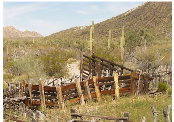
Figure 26: Post and board fencing made from widely spaced timber posts and dimensional lumber rails. This is the least common type of fencing at Bates Well Ranch and is mostly associated with the cattle chute, which is of similar construction. Photo: Randall Skeirik, NPS
