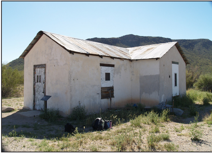
Figure 14: The Main House at Bates Well Ranch. The house was assembled from two separate buildings that were moved to the ranch from the nearby Growler Mine site after the mine closed. Photo: Joe Tuomey, NPS
