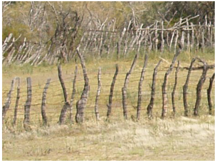
Figure 24: A more typical barbed wire fence made with mesquite posts strung with barbed wire. As with other fence types that use mesquite posts, many of the posts have rotted off below grade causing the fence to collapse. Photo: Randall Skeirik, NPS
