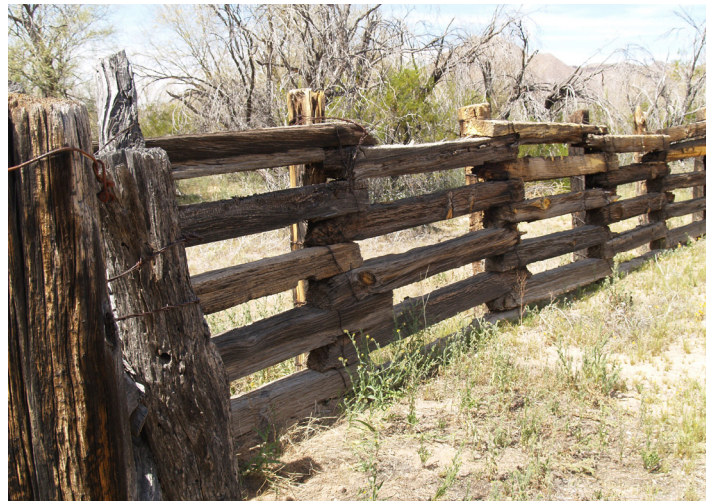
Figure 21: Stacked timber fencing made from reused railroad ties utilized material more efficiently than the stockade type. Although inherently more stable, the overlapping section of each run is supported by a post, and like the stockade fence, these posts have rotted below grade allowing sections to fall. Photo: Randall Skeirik, NPS
