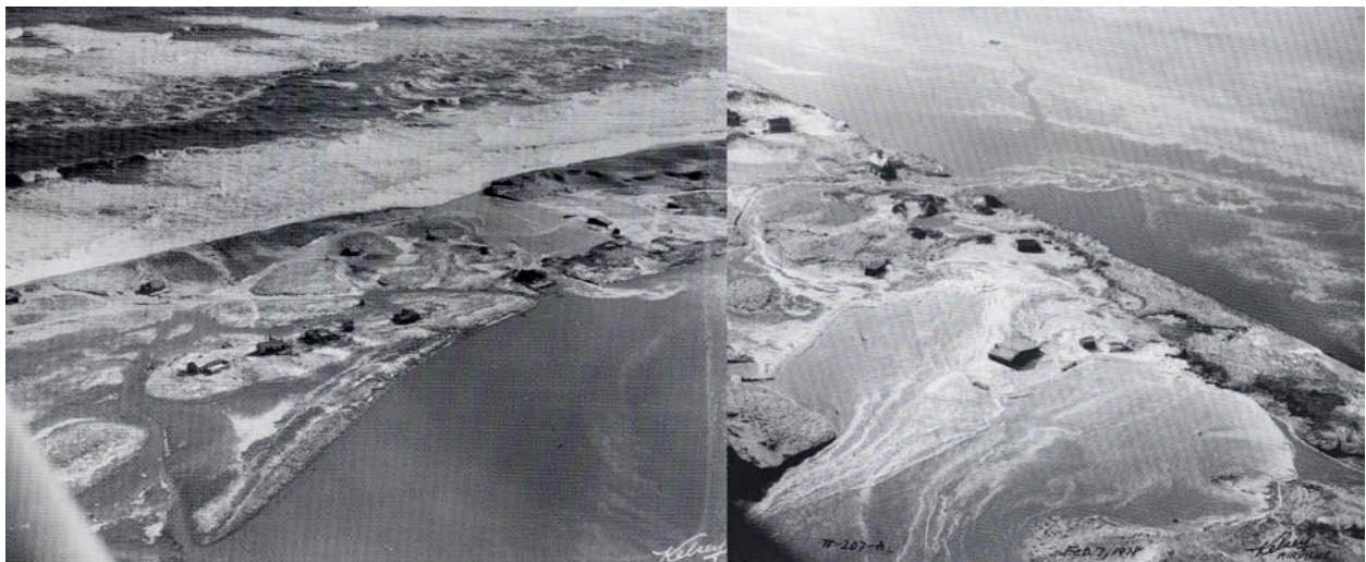
Figure 10. Photos of Chatham's North Village after the storm of 1978. (from Higgins, Frances 2004, Drifting Memories: Nauset Beach Camps on Cape Cod . Lower Cape Publishing, Orleans MA). Photos by Richard Kelsey. Courtesy of Warren Quinn.
