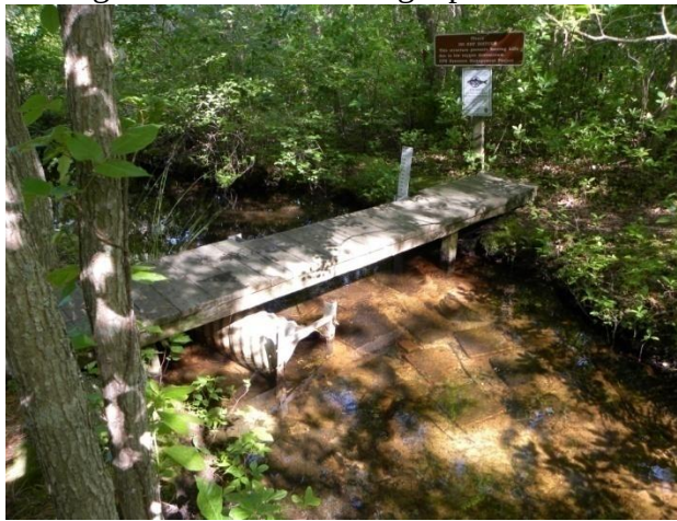
Herring Pond Outlet Culvert and Bridge
