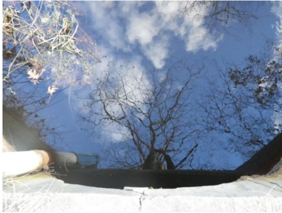
Looking down at the Bound Brook Culvert
