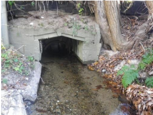
Old Kings Highway Culvert
