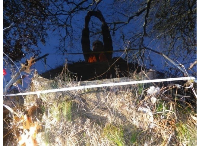
Looking down at the Pole Dike Culvert
