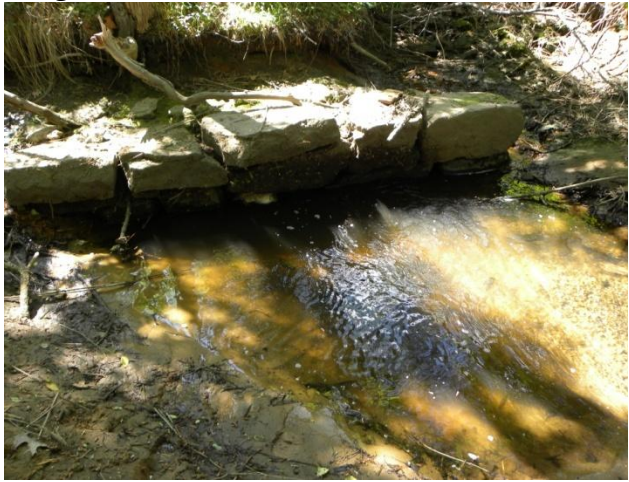
Fresh Brook Culvert
