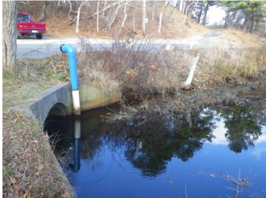
Bound Brook Culvert
