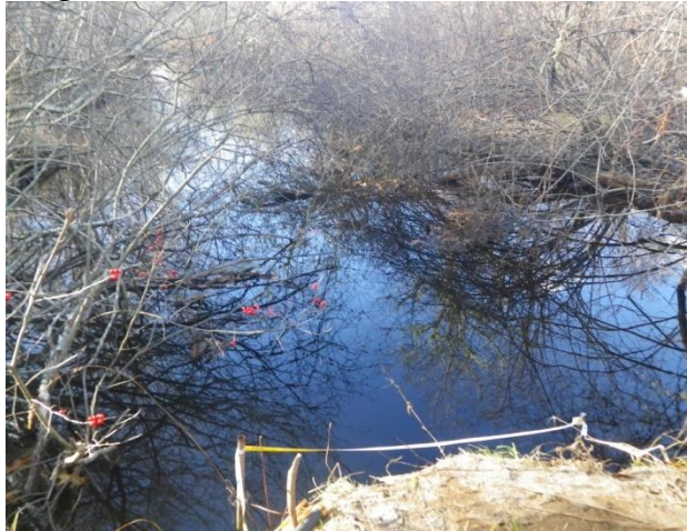
Pole Dike Site looking downstream from the culvert.
