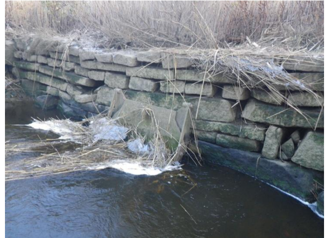
Pamet River Post Office Culvert
