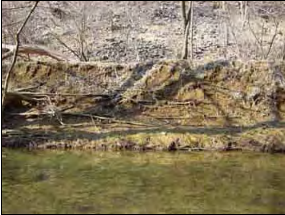
Erosion Location 15 December 20, 2003)
