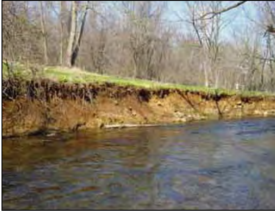
Erosion Location 35 (April 4, 2004)
