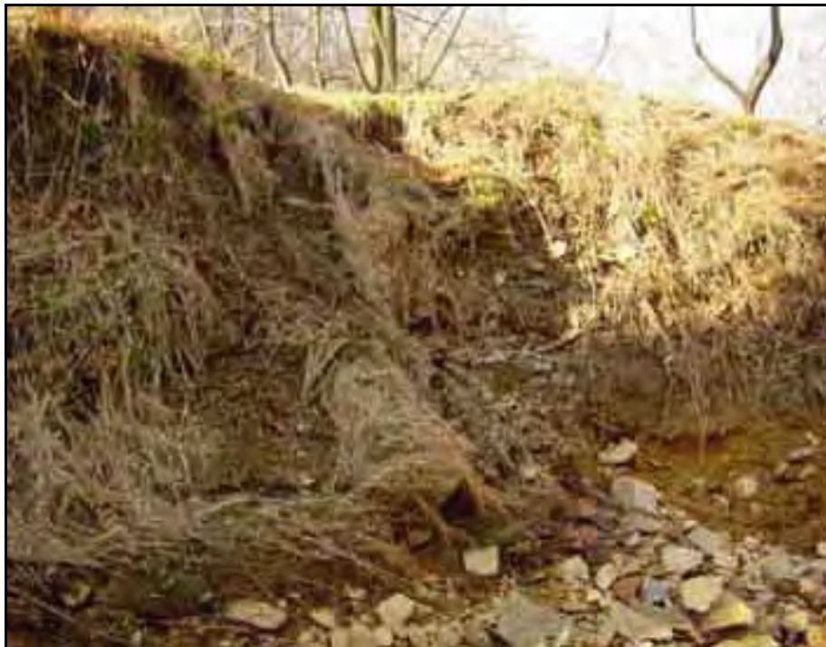
Erosion Location 12 (December 13, 2003)
