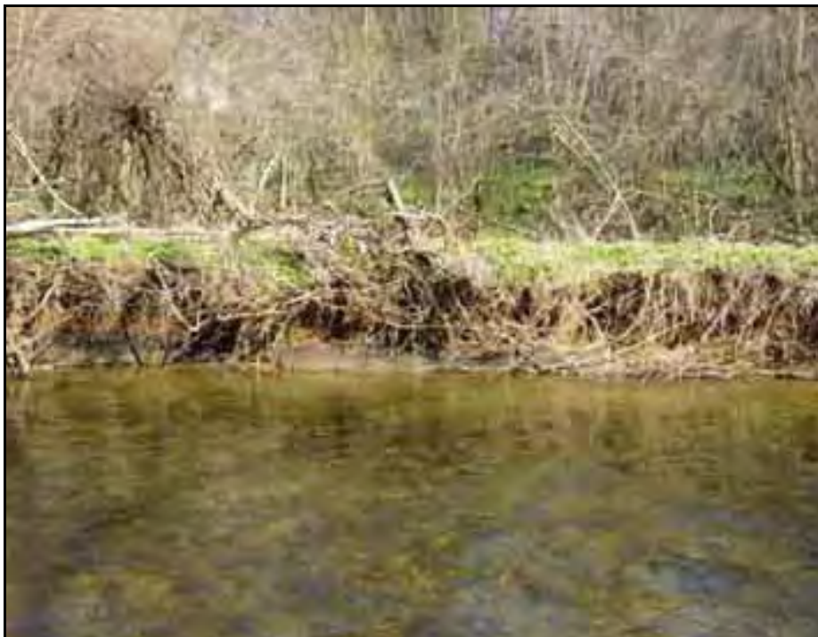
Erosion Location 36 (April 4, 2004)
