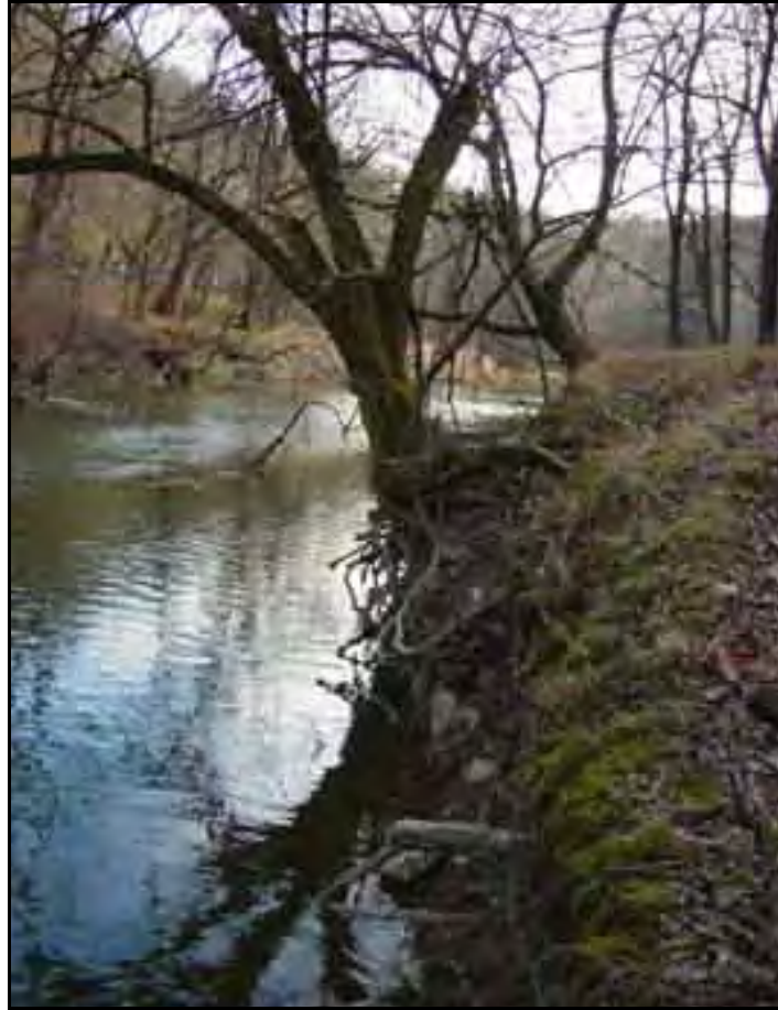
Erosion Location 7 (December 13, 2003)
