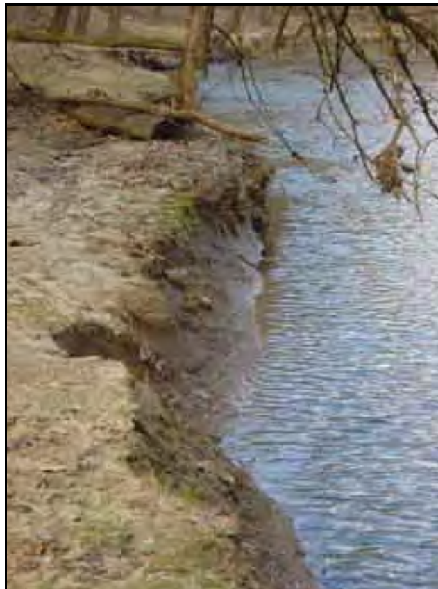
Erosion Location 6 (December 13, 2003)
