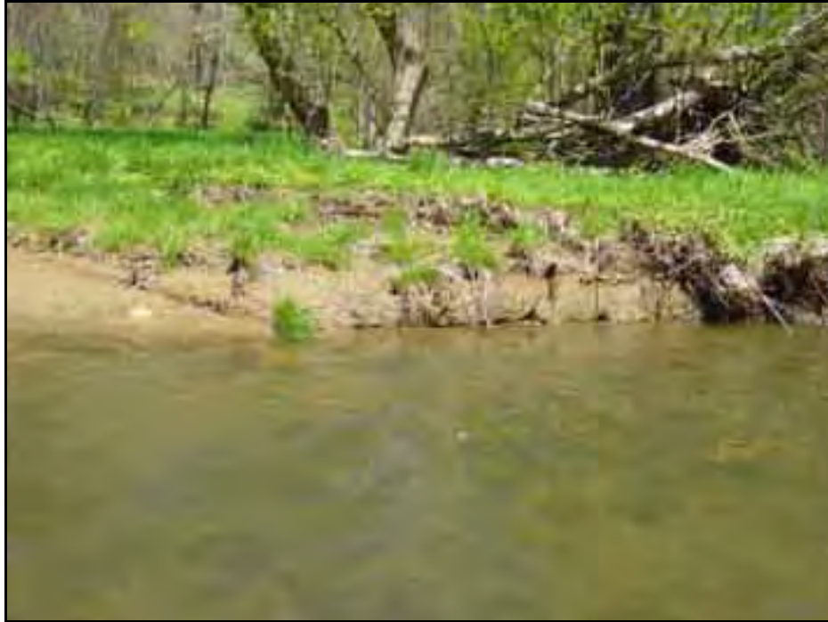
Erosion Location 37 (April 4, 2004)
