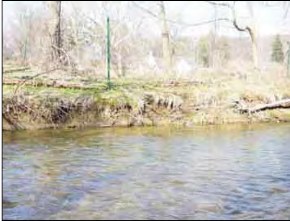
Erosion Location 27 (February 20, 2004)
