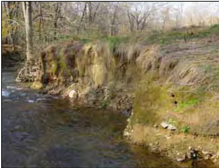
Erosion Location 4A (November 8, 2003)
