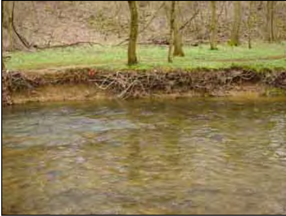
Erosion Location 33 (April 3, 2004)
