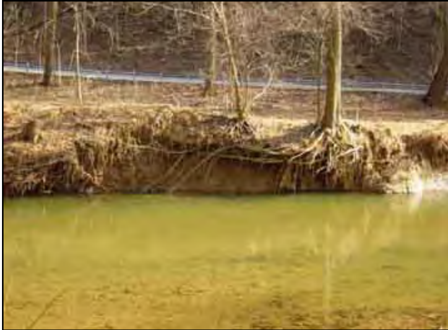
Erosion Location 13 (December 13, 2003)
