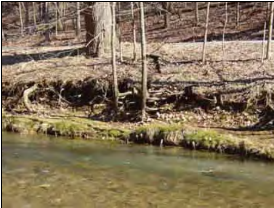
Erosion Location 16 (December 20, 2003)
