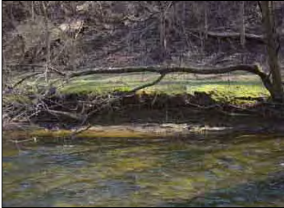
Erosion Location 29 (February 20, 2004)
