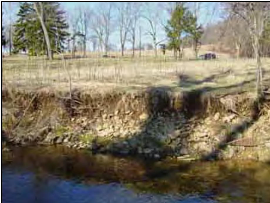
Erosion Location 22 (February 20, 2004)
