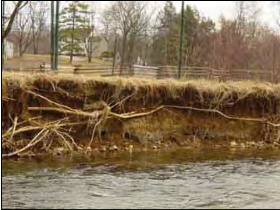
Erosion Location 21 (December 20, 2003)
