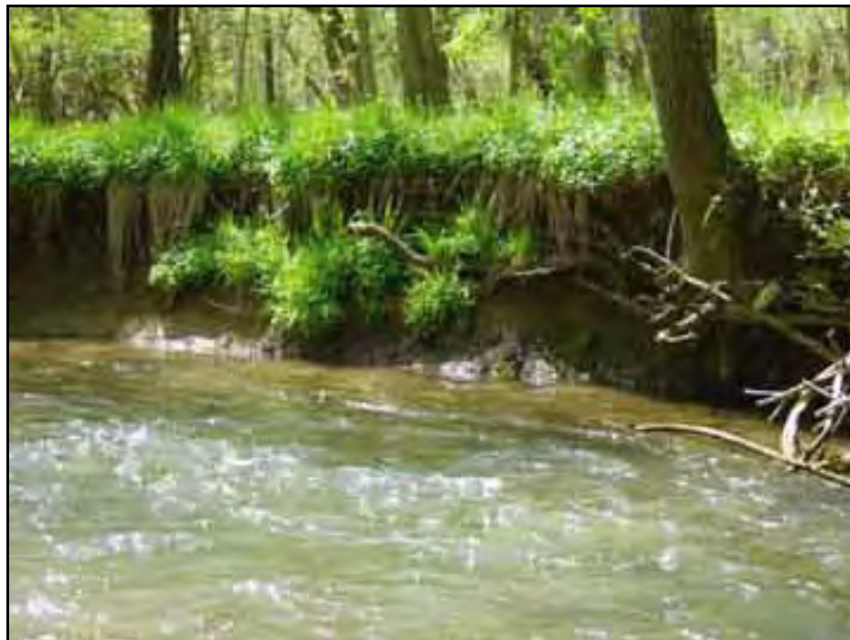
Erosion Location 38 (April 4, 2004)
