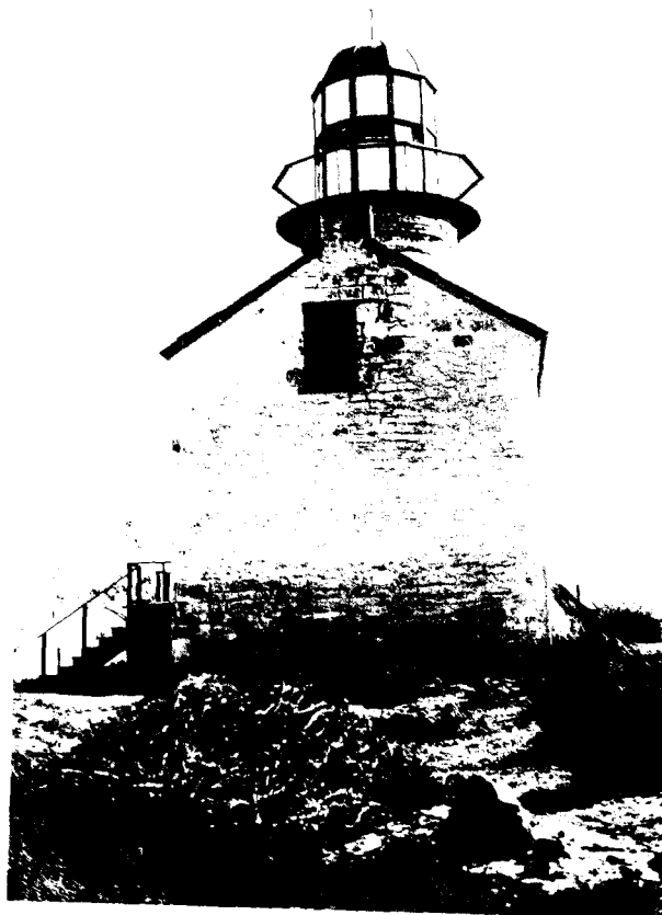
North elevation of Lighthouse. Outside stairs to basement may be seen at lower right-hand corner of building.
