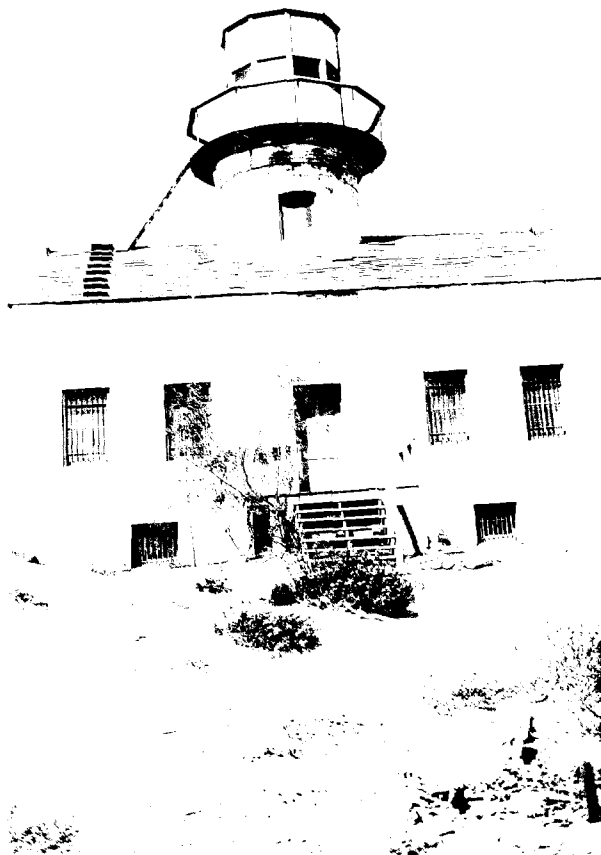
East elevation of "Old Spanish Lighthouse". The wooden porch and steps should be replaced by stone steps. In the foreground are remnants of the concrete watershed which once covered the entire front yard.
