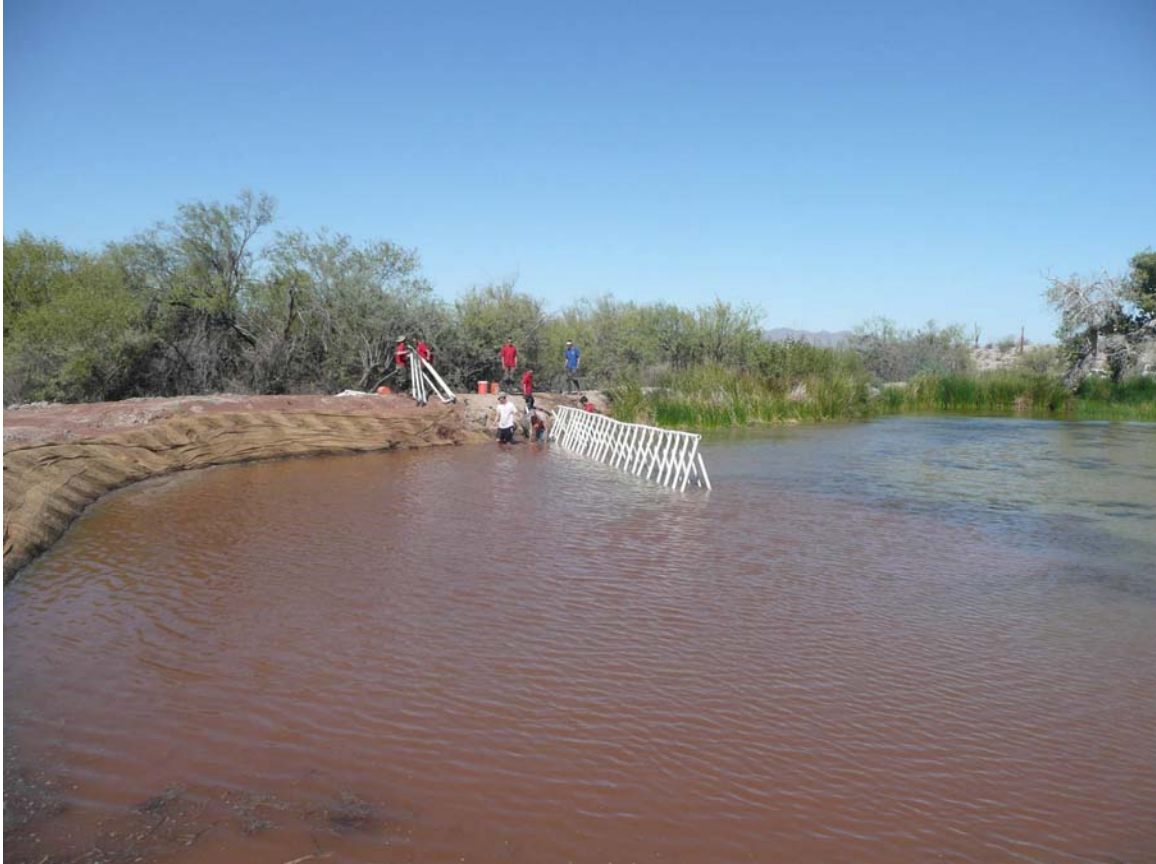
Figure 17. Quitobaquito Pond, September 23, 2009. Removing the last parts of the temporary coffer dam. Renovated/sealed southeast corner is left of the white dam frame.
