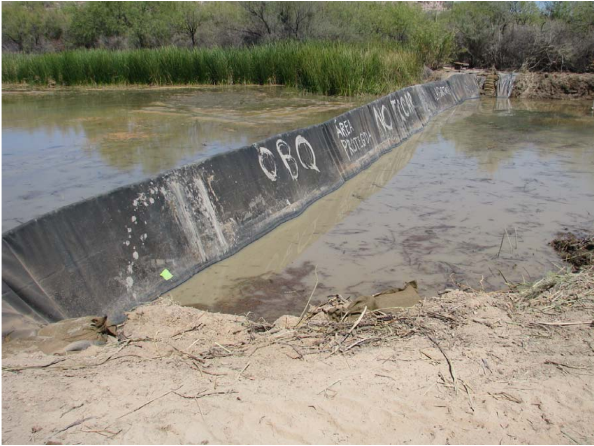
Figure 9. Completed coffer dam, Quitobaquito Pond, August 18, 2009.
