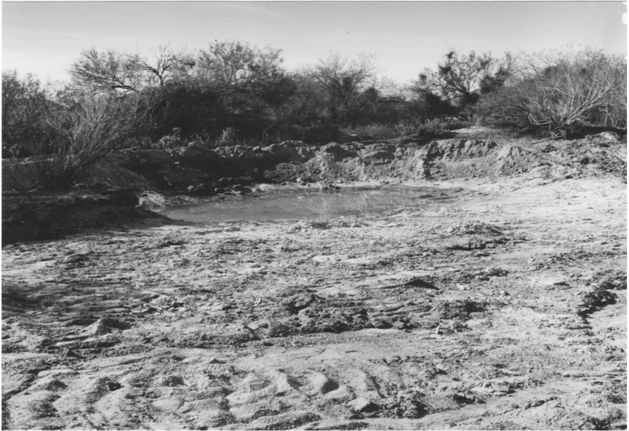
Figure 18. Quitobaquito Pond, view from center of pond southeast, into southeast corner, January 1962. Photograph taken during major 1962 renovation. NPS File photo, W.F. Steenburg.
