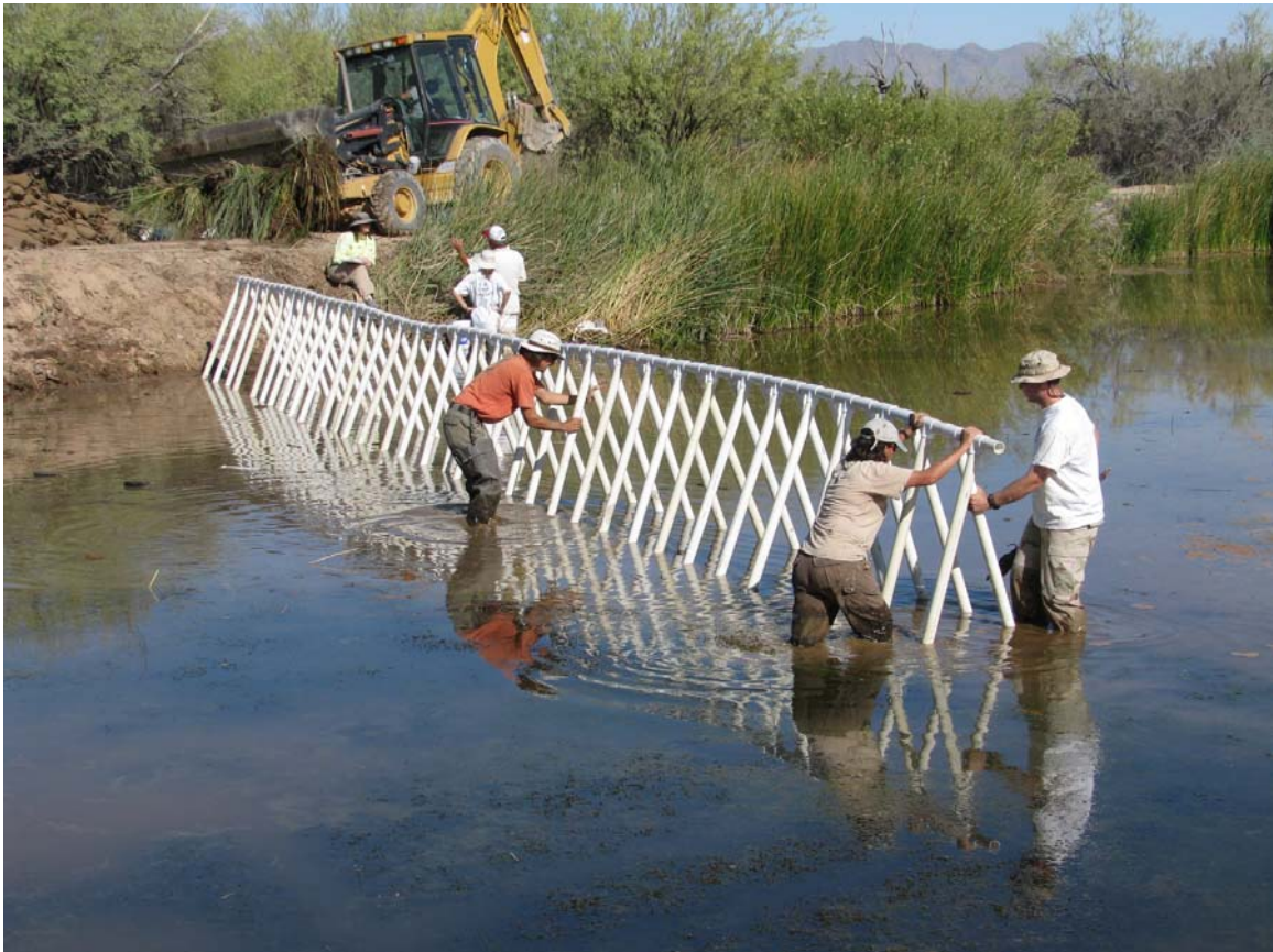
Figure 8. Assembling the frame for the coffer dam, Quitobaquito Pond, August 18, 2009.
