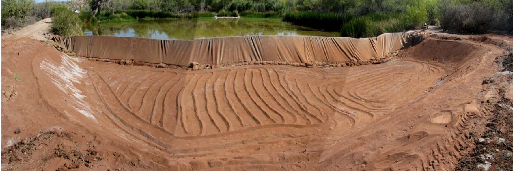
Figure 15. Southeast corner of Quitobaquito Pond, renovated and sealed with a compacted mixture of clean earth and bentonite. August 28, 2009.
