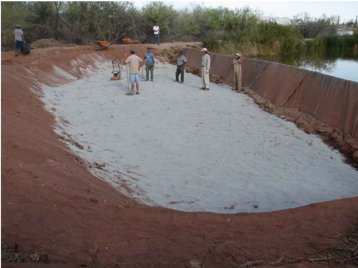
Figure 14. Layer of bentonite (white) spread on the pond bottom, awaiting overlayer of red fill material prior to compacting. The former deep well area was in the lower left corner of this view. August 28, 2009.
