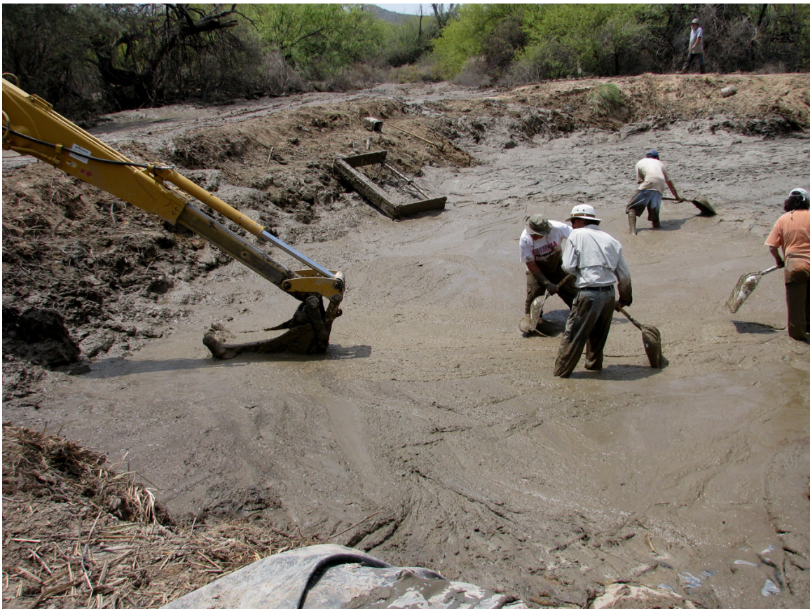
Figure 12. Removing mud and organic detritus from the southeast corner of Quitobaquito Pond. August 21, 2009.
