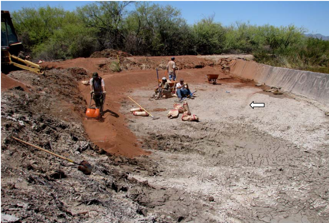
Figure 13. Compacting bentonite-enriched fill against exposed inner face of the retaining berm. The pre-existing clay pond bottom is visible as a grey floor, drying out. The white arrow points to "the trough," visible as a faint dark linear feature fading into the damp area at the base of the coffer dam. August 25, 2009.
