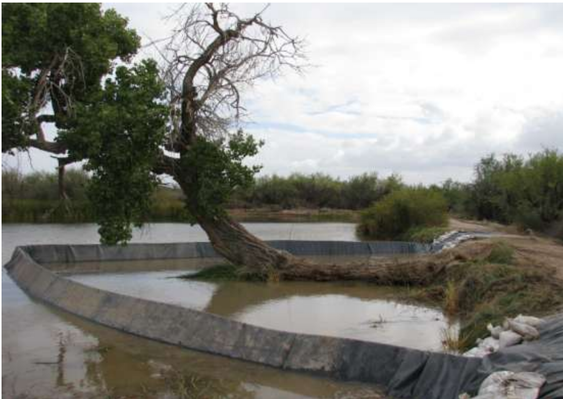
Figure 4. Cofferdam in place. October 19, 2010.
