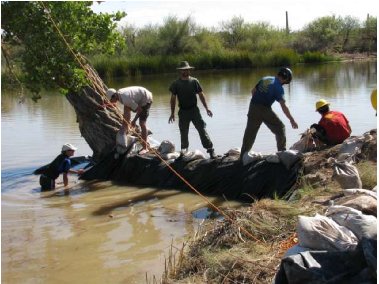
Figure 7. Sealing tree with pond liner. October 26, 2010.
