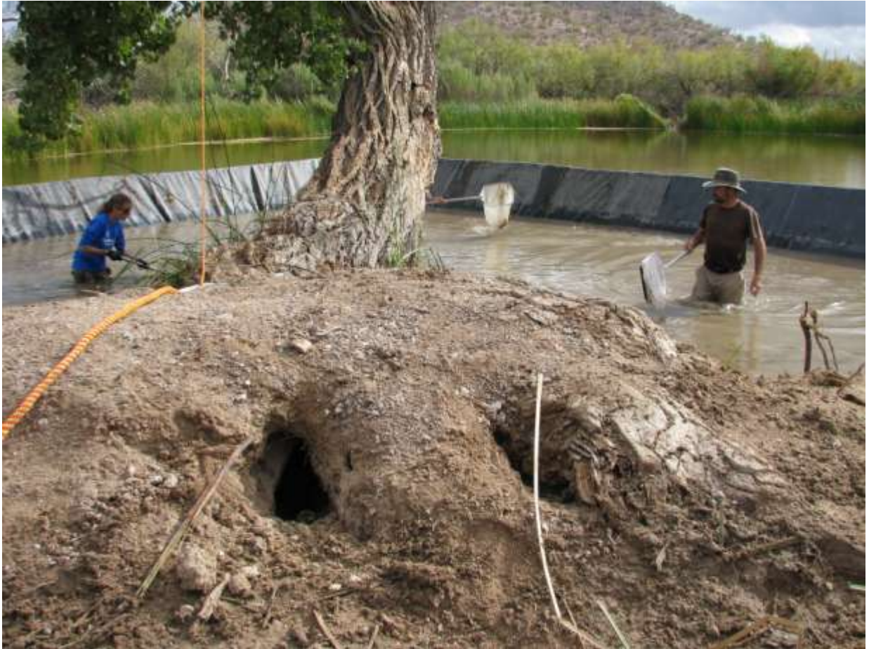
Figure 9. Holes at base of cottonwood, among roots and extending into berm. Eventually found to extend 5 feet down and toward pond. October 20, 2010.
