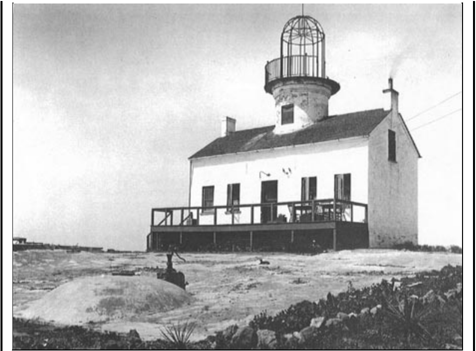
Figure 4: Point Loma Lighthouse used for military housing, ca. 1917. Rainshed pavement and cistern exist but lens and illumination systems are missing (National Park Service photograph from historical collection of Title Insurance and Trust Company, San Diego).
