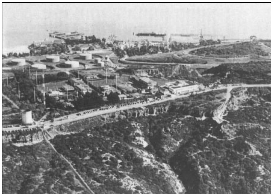
Figure 23: Ca. 1936-1941 Photograph of Naval Radio Station and Sound Research Laboratory (foreground) which received the first radio message of the Pearl Harbor
