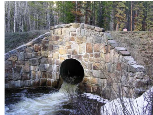
Figure 4. Timber Creek Culvert Rock Work Photo: Amanda Jeter (2008)
