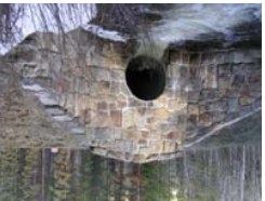
Timber Creek Culvert
