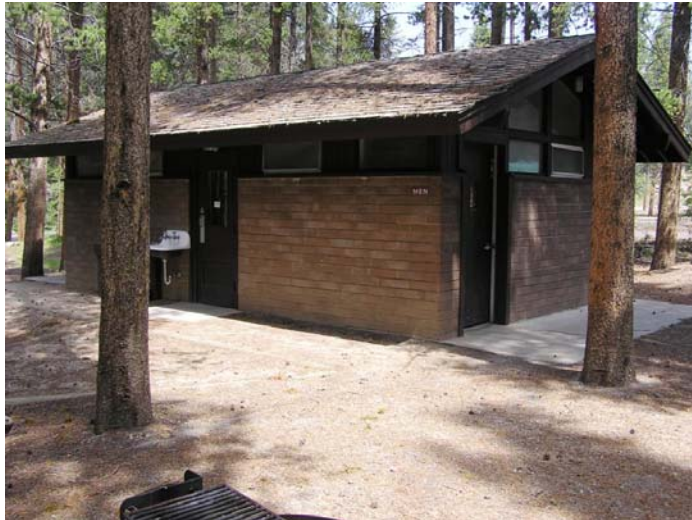
Figure 8. Timber Creek Comfort Station, c. 1963. Photo: Amanda Jeter (2008)
