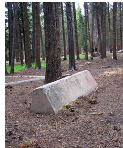
Figure 21. Remnant Mission 66 Era concrete curb in Timber Creek. Photo: Amanda Jeter (2008)
