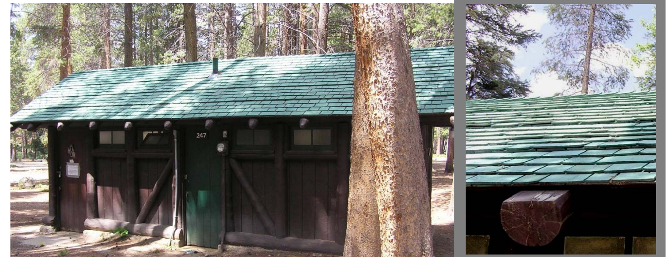
Figure 7. Timber Creek Comfort Station #247, c. 1940 & Shingle Detail. Photo: Amanda Jeter (2008)
