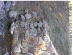
Timber Creek Culvert 3
