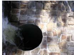
Timber Creek Culvert 2
