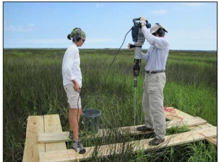
Figure 8. NPS staff installing a RSET monitoring station at Timucuan Ecological and Historic Preserve.
