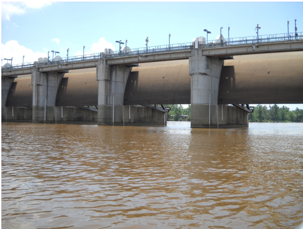
Figure 1. The Saltwater Barrier of the Neches River during above-normal flow conditions. Photograph by Joe Meiman, May 14, 2009. Note open gates to accommodate high discharge of the Neches River and elevated turbidity at this time; maximum flow was 4,450 cfs on this date.
