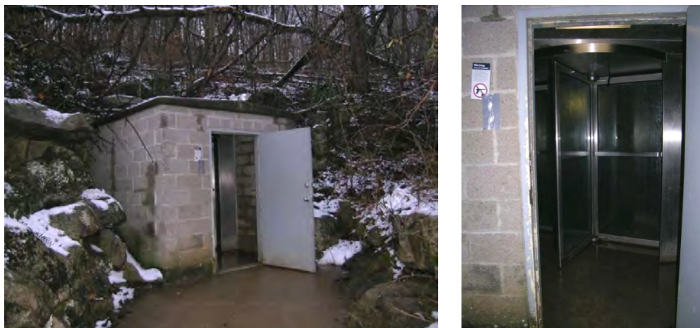
Figure 3. Blockhouse at the Frozen Niagara Entrance to Mammoth Cave. Note the airtight, rotating door in the rightmost image that prevents air from pouring in while the outer door is open but still permits visitors to pass.
