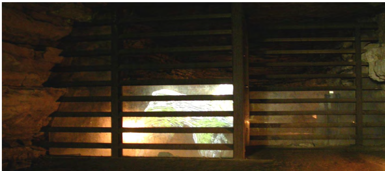
Figure 1. Current gate/Plexiglas configuration at the Historic Entrance to Mammoth Cave. For the previous configuration, there was no Plexiglas paneling in place. In the winter, surface air was free to pour into that part of the cave unabated.
