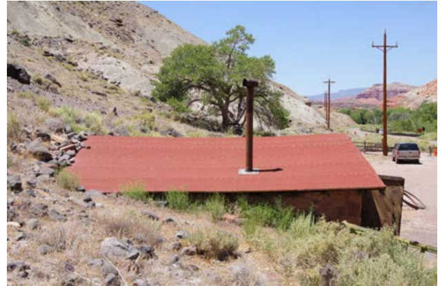
Shed following Repairs
