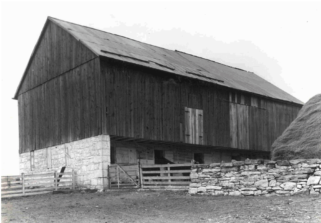
Poffenberger barn as documented by Thomas Waterman of the Historic American Building Survey in 1940. (ANTI 1940)
