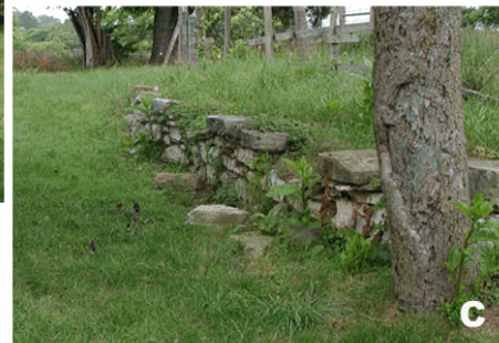
A) Joseph Poffenberger farmhouse with addition; B) Detail of original stone steps to front porch; C) Limestone wall behind ell addition. (CLP 2006).
