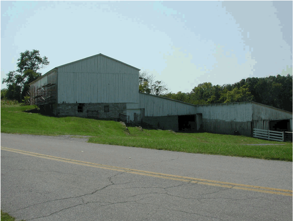
Contemporary view of the Miller barn, showing altered roof pitch and livestock additions. Photograph by author, September 2003.
