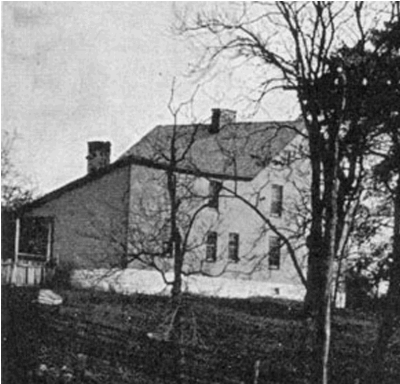
1906 view of the Miller farmhouse, showing flounder roof kitchen addition with integral porch. Central chimney is clearly visible on the main block. Reprinted from Oliver T. Reilly, The Battlefield of Antietam (Sharpsburg, MD: Oliver T. Reilly, 1906).
