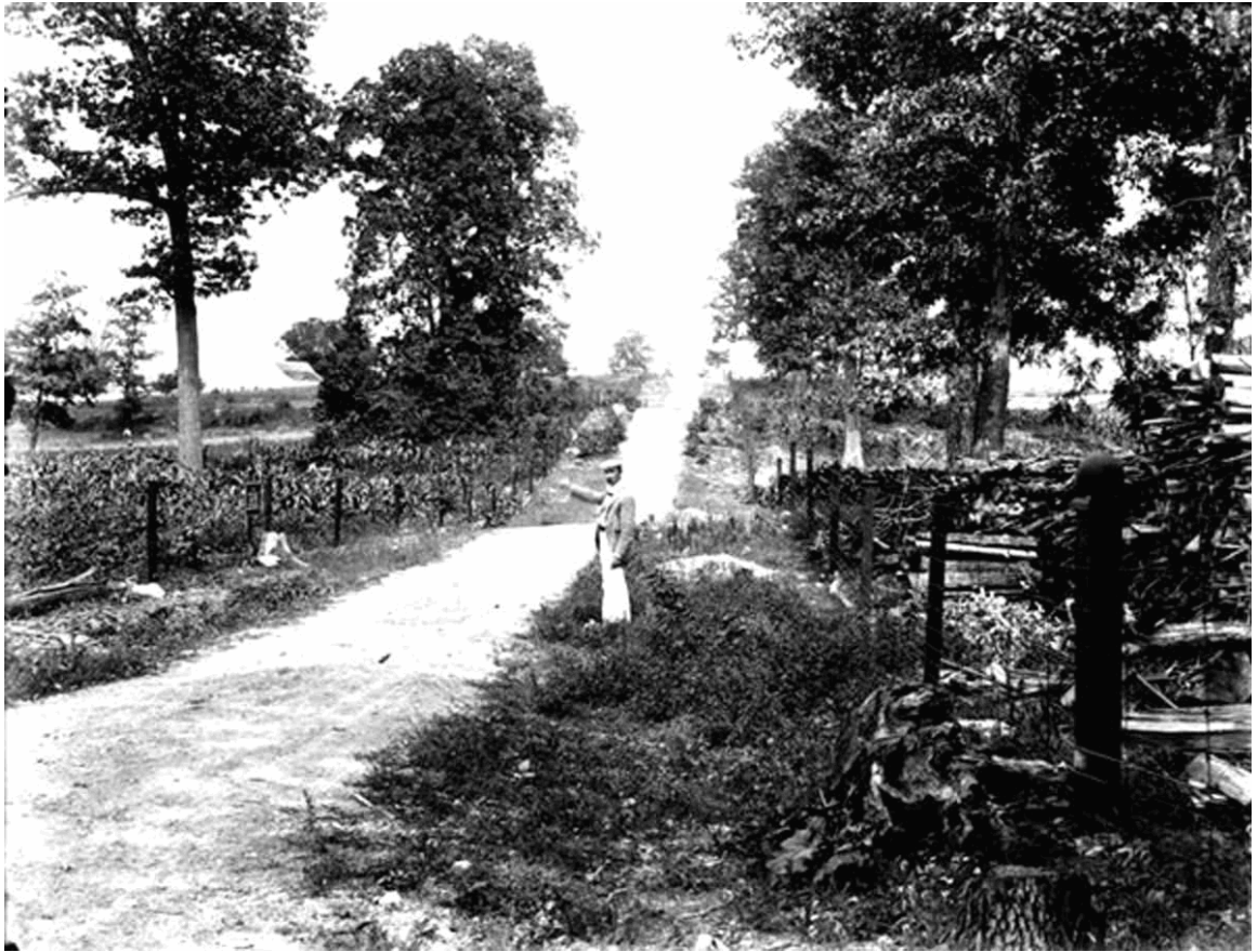
Looking east along Mansfield Avenue north of the Miller Farm. The North Woods are visible in this circa 1900 photo, as is the War Department-era fencing. Reprinted from http://www.nps.gov/anti/gallery.htm .
