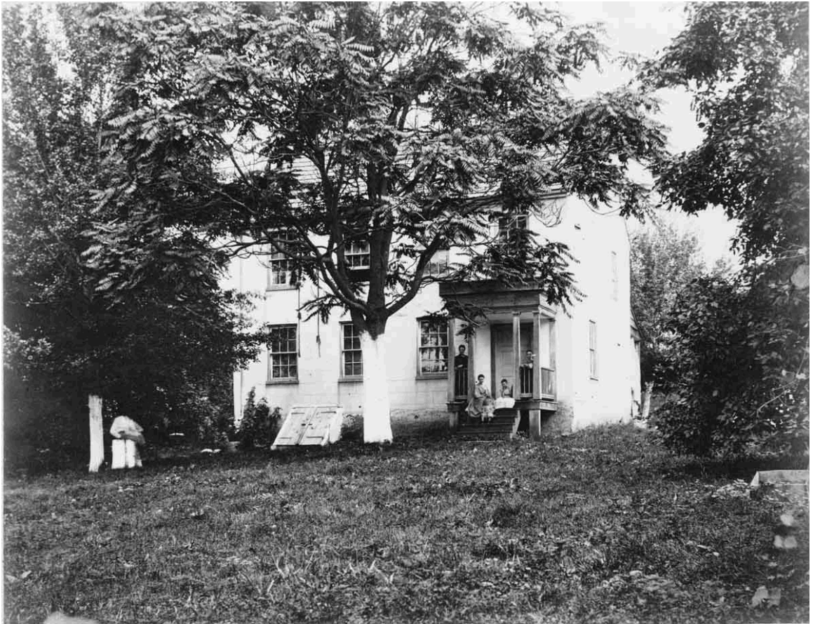
Circa 1862 view of Miller farmhouse showing Greek Revival porch and scored stucco made to resemble ashlar blocks. Reprinted from http://lcweb2.loc.gov/cgi-bin/query/r?pp/ils:@field(NUMBER+@band(cph+3c04417)) .
