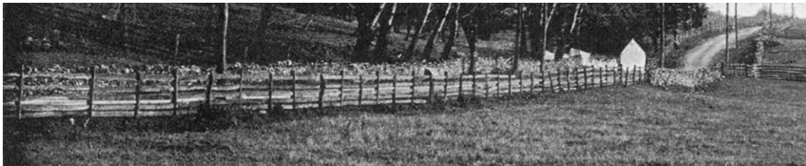
1906 photograph showing various types of fencing employed along the Hagerstown Pike. Reprinted from Reilly.
