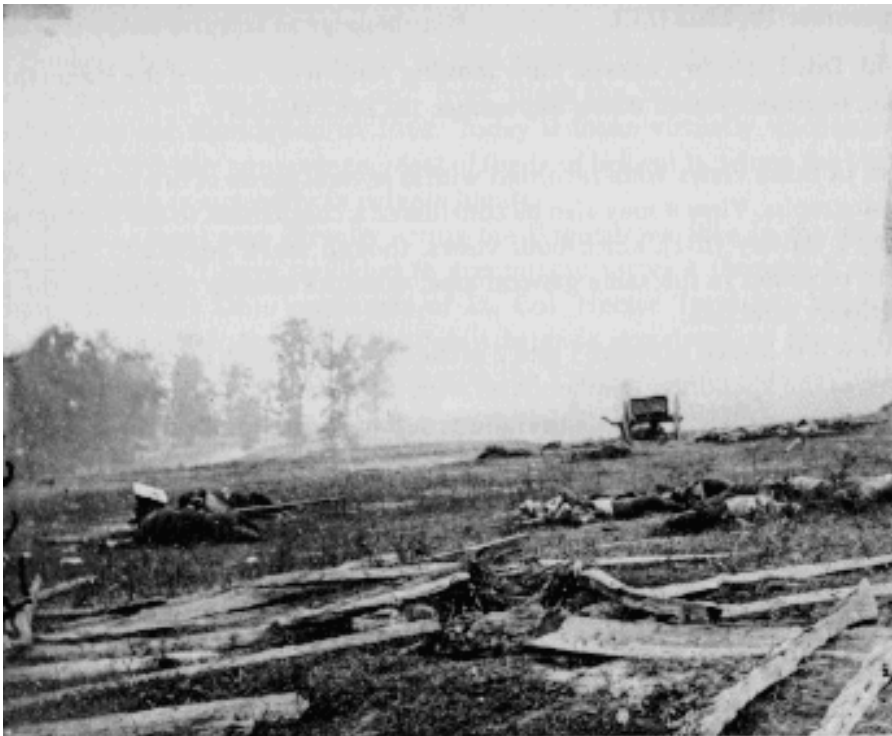
Devastation at the western corner of the Mumma Farmstead, 19 September 1862. This area is now the site of the Maryland Monument Park. Library of Congress, Gardner stereophotograph #568.
