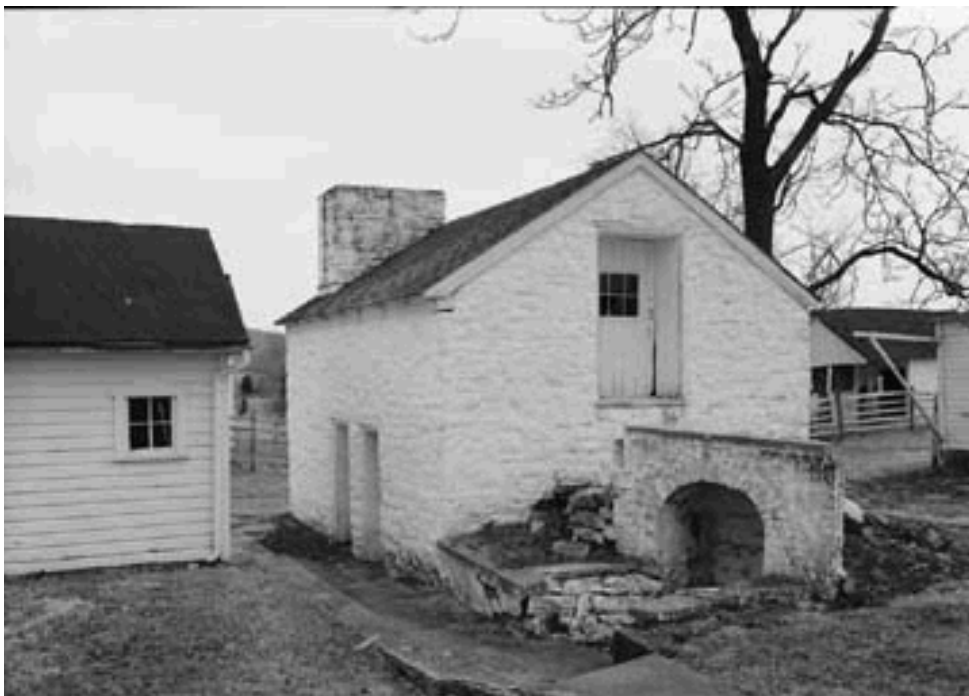
Mumma spring (foreground) and stone springhouse. Historic American Buildings Survey photograph, 1988.
