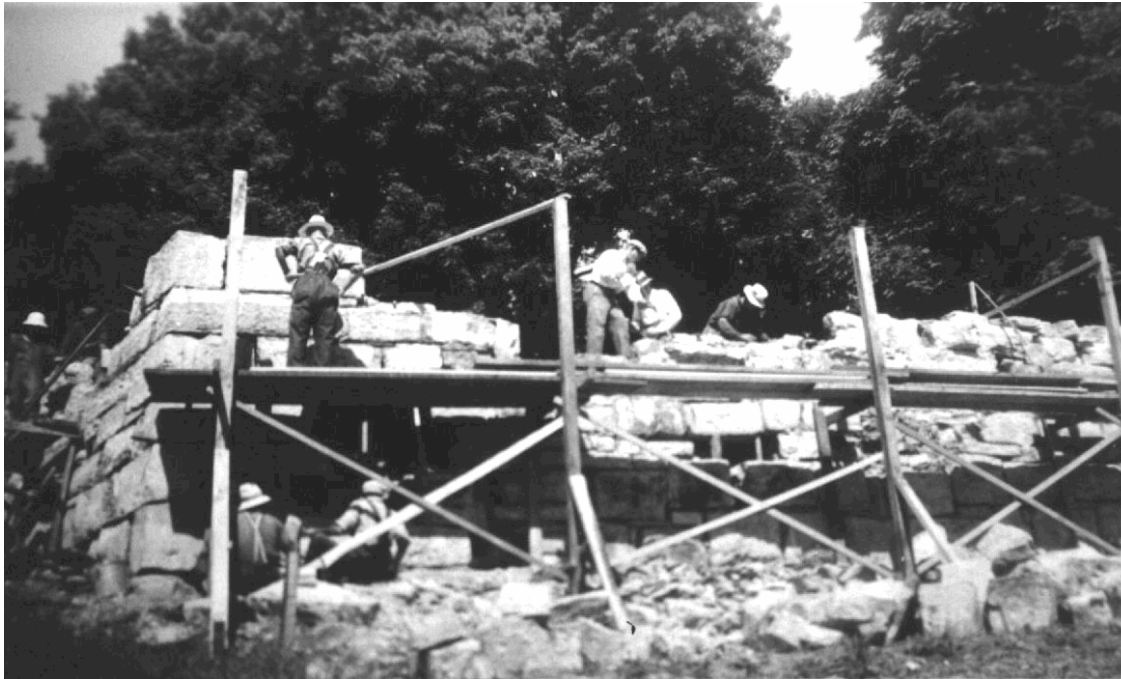
Exterior view of the WPA wall project, 1939. (National Archives)
