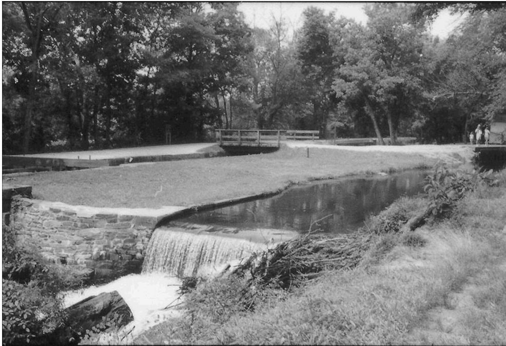
Lock 19 bypass flume (2000).
