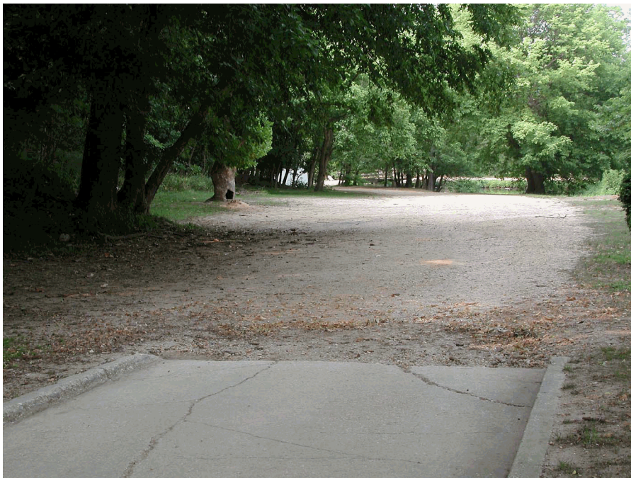
View of access lane behind tavern looking south towards Lock 19. Note change in material from concrete to gravel/dirt.
