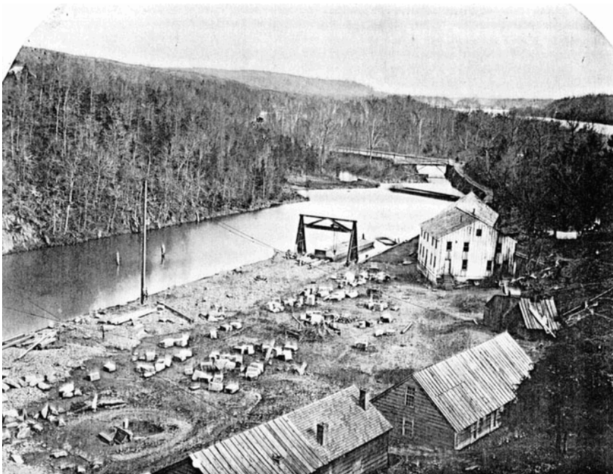
View below Lock 17 looking south towards the stopgate. Construction and buildings relate to the aqueduct (Circa 1862).
