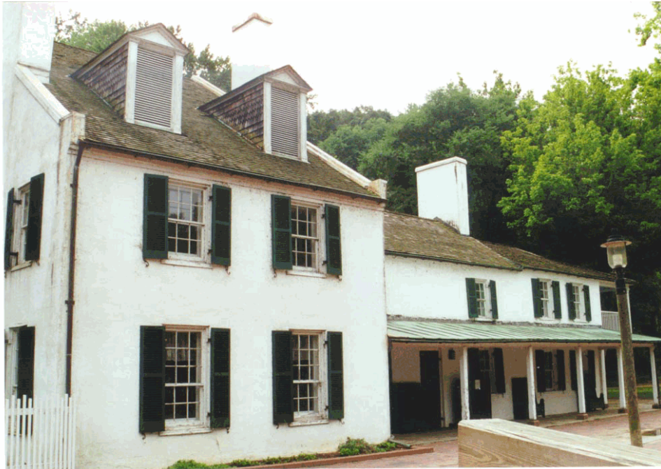
The tavern, west façade (2000).
