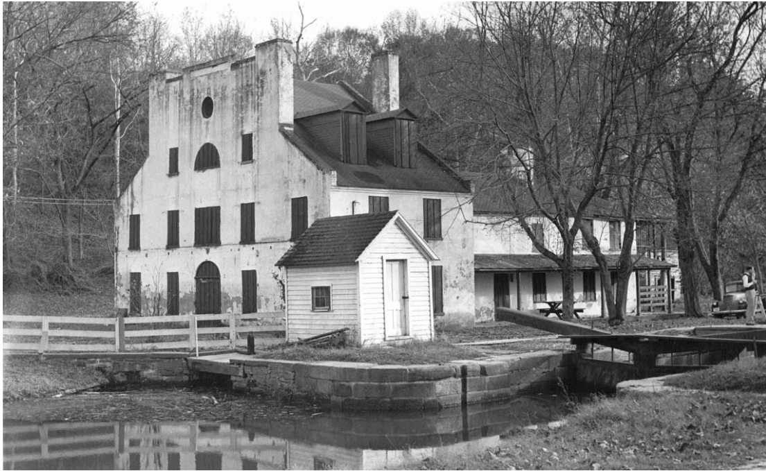
The canal and lock have been repaired but the tavern is closed and derelict (circa 1946).
