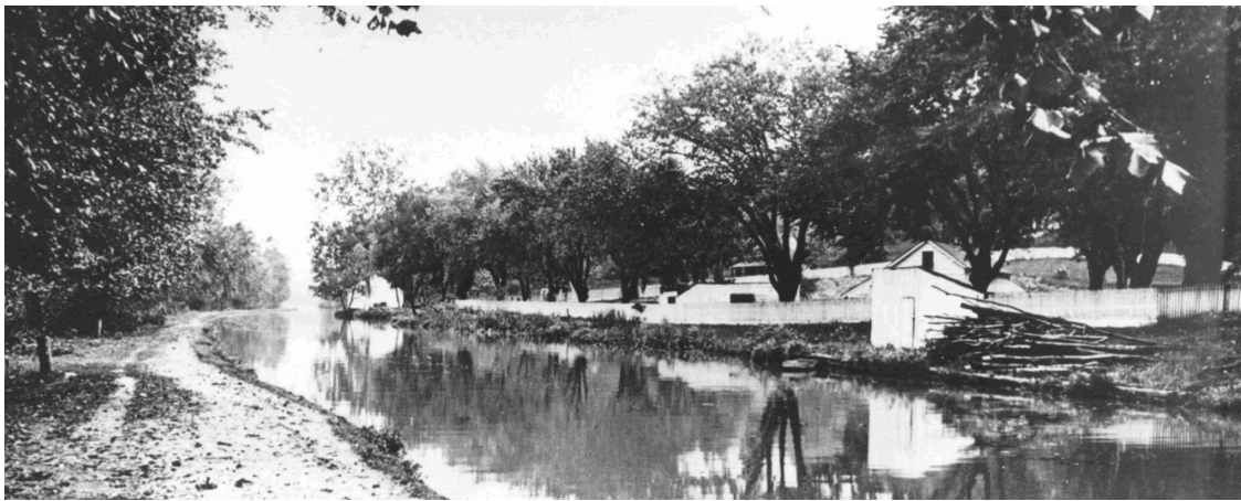
View north of the tavern. The picket fence surrounds the Army Corps of Engineers property. The building located further down the canal is the C&O Canal carpenter's shop (Circa 1900).
