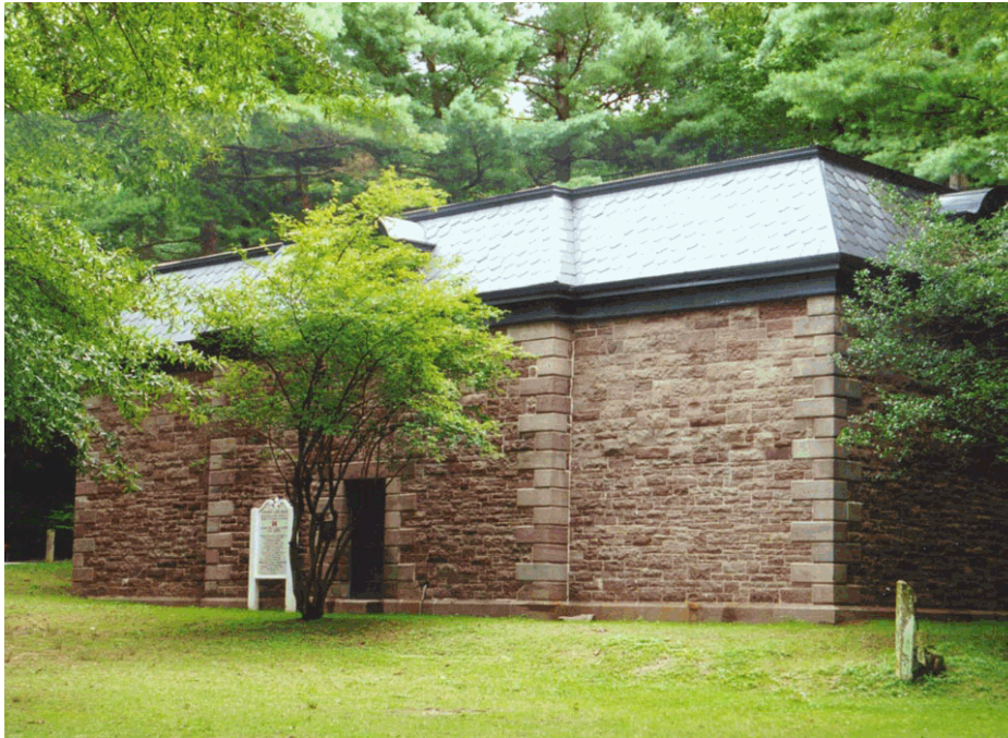
Nineteenth-century gatehouse, Washington Aqueduct. Note concrete mile-marker in lower right (2000).
