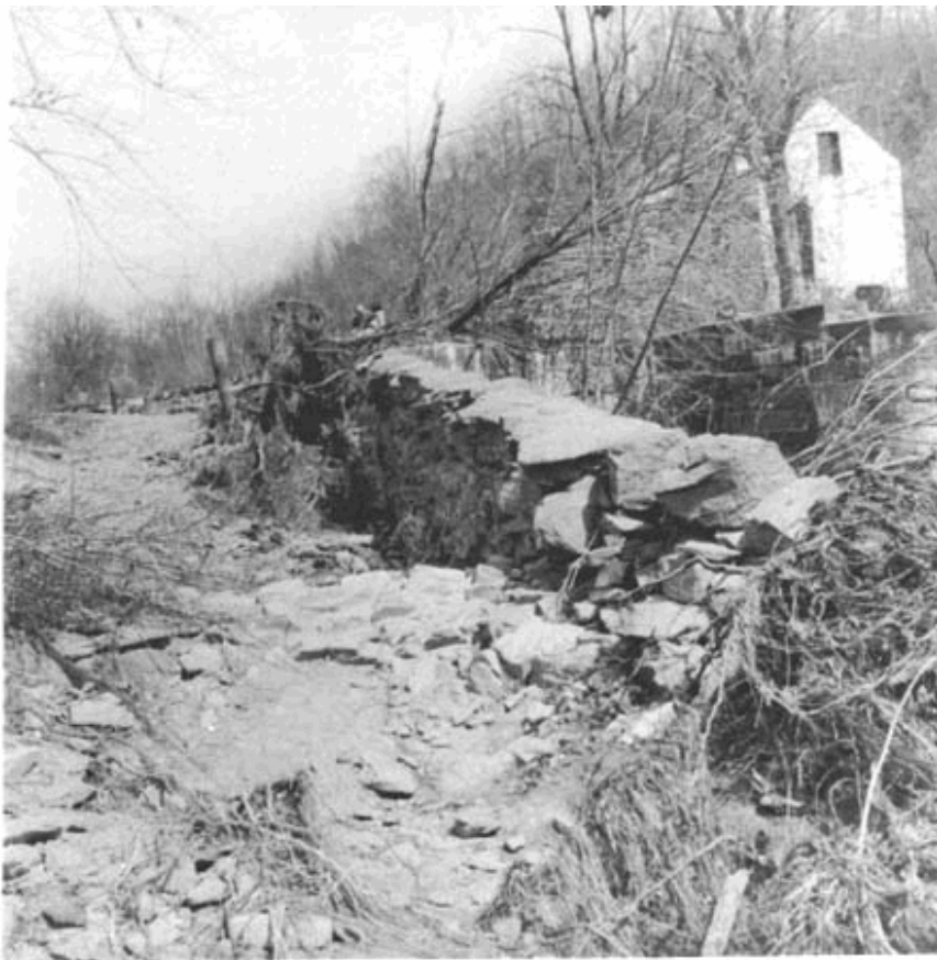
1936 flood damage at Lock 18.
