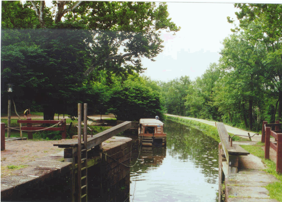
Lock 20, looking south. Note replica canal boat heading for lock (2000).
