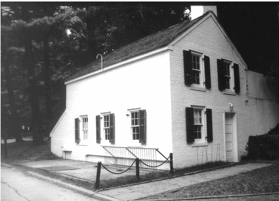
CCC constructed pump house located northeast of the tavern (2000).
