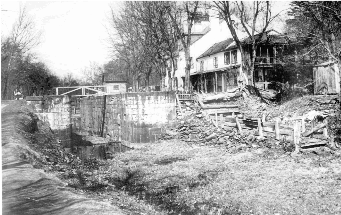
The tavern and Lock 20 after the 1936 flood. The CCC repaired this damage after the NPS purchased the canal.
