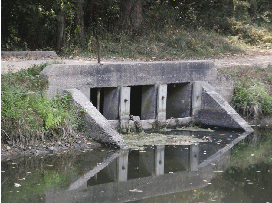
Concrete waste weir inflow on upper level of canal, with towpath crossing it. Waste weir was built c. 1909. Before that, there seems to have been an informal overflow a little farther upstream. (2002, M. Gerdes)
