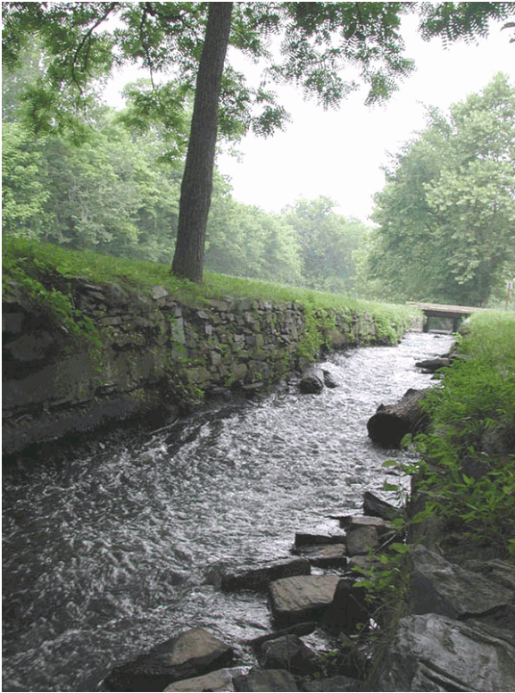
Bypass flume. Water cascades on riprap "tumble" and banks are secured with dry masonry. Feature is discussed in Buildings and structures." (2002, M. Gerdes)
