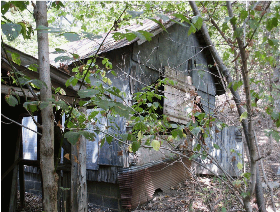
Tin-sided one-car garage still standing. Some of the dilapidated structures have handhewn beams. (2002, M. Gerdes)
