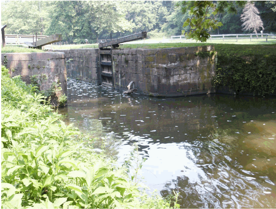
Lock walls, including lock extension walls and headwalls, seen from lower level. Fence at upper right encloses grass field by Pennyfield House. (2002, M. Gerdes)
