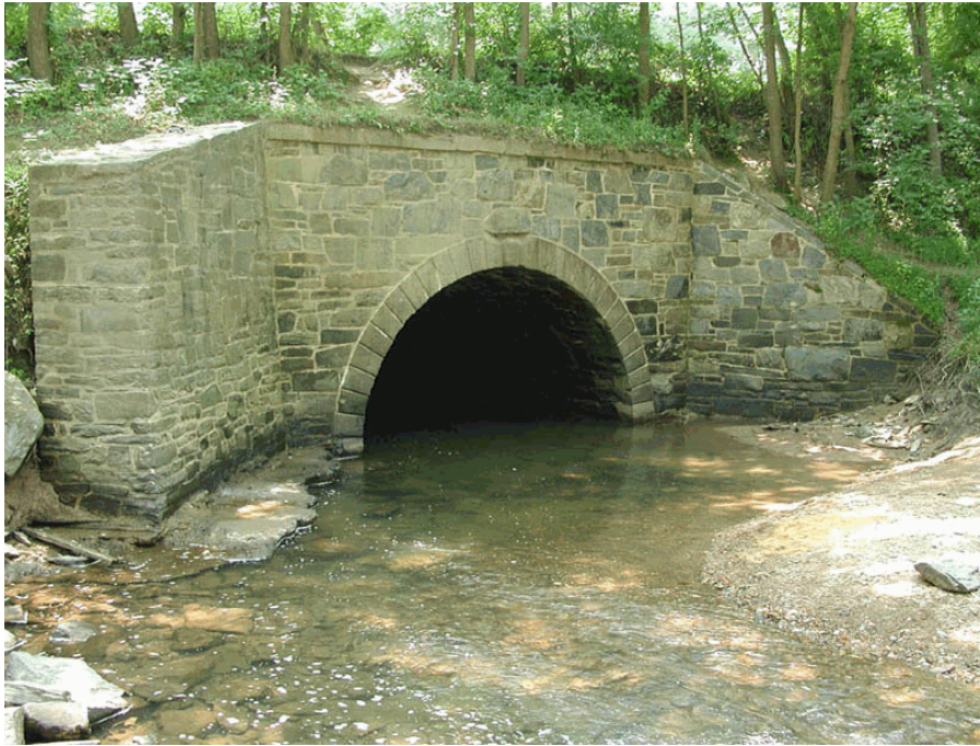
Headwalls of Muddy Branch culvert on inland side. (2002, M. Gerdes)
