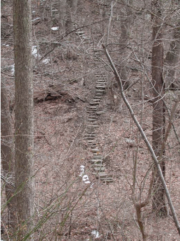
Stone slabs set into slope create staircase east of Pennyfield House. (2003, J. Earley)
