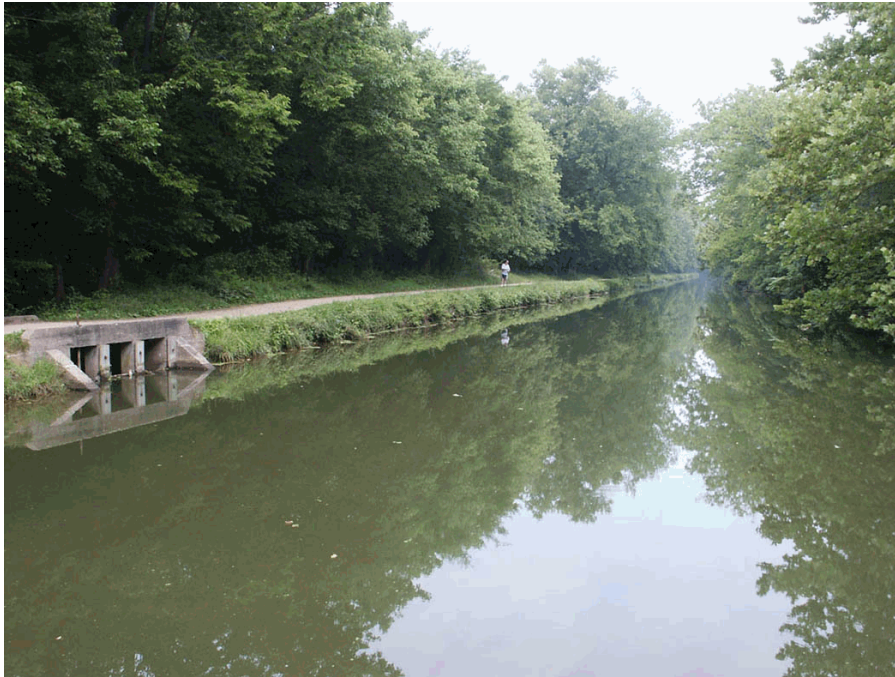
Linear character of the canal, looking west. Structure on left is waste weir inflow. (2002, M. Gerdes)
