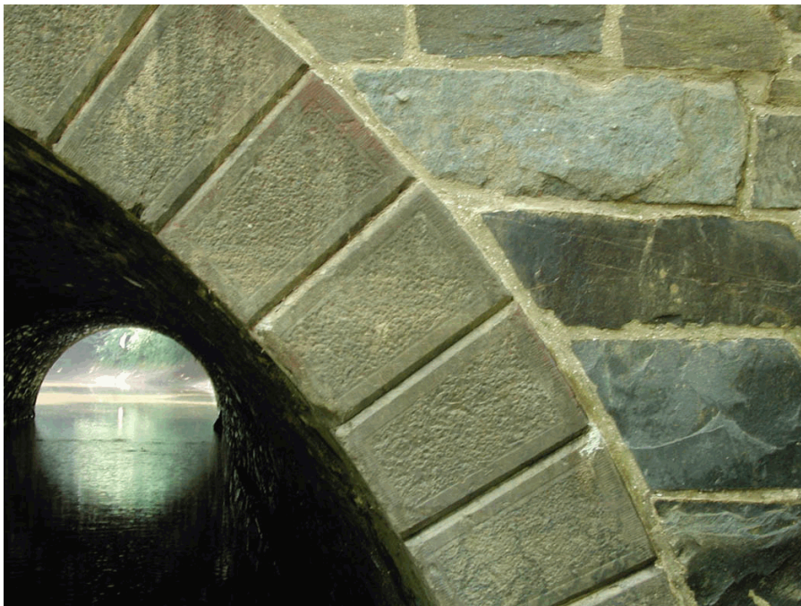
Closeup view of stonework of arch ringstones. View through culvert to other side. (2002, M. Gerdes)
