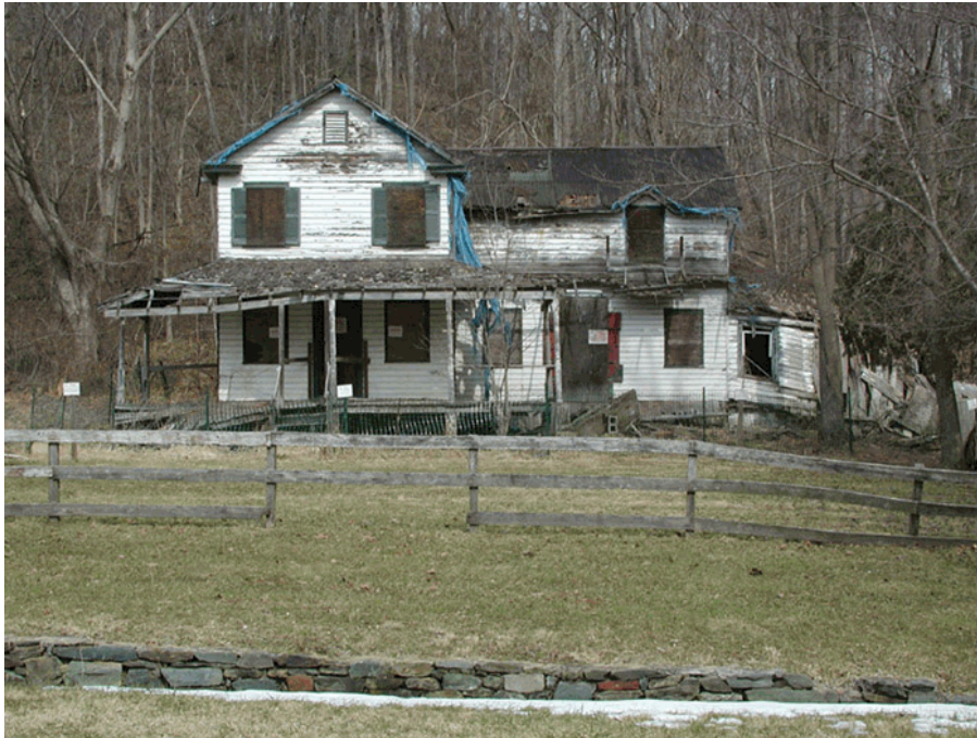
Pennyfield House. Stonework in lower part of view is bypass flume retaining wall. (2003, J. Earley)
