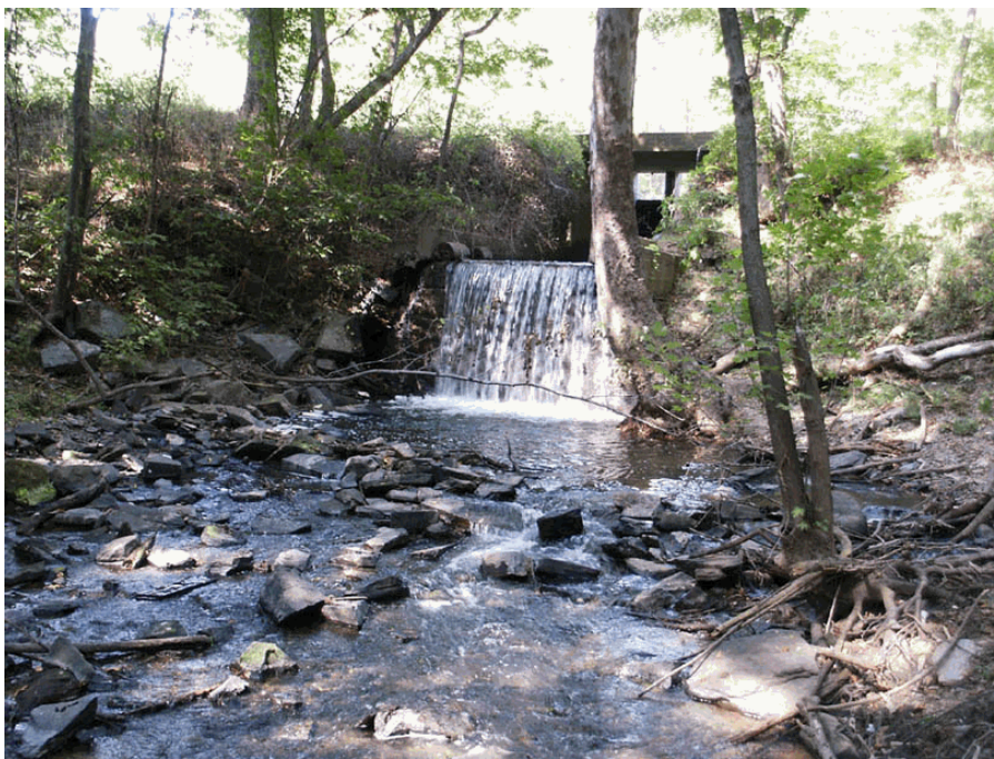
Overflowing water from the canal upper level through the waste weir has carved a small stream in the floodplain. (2002, M. Gerdes)
