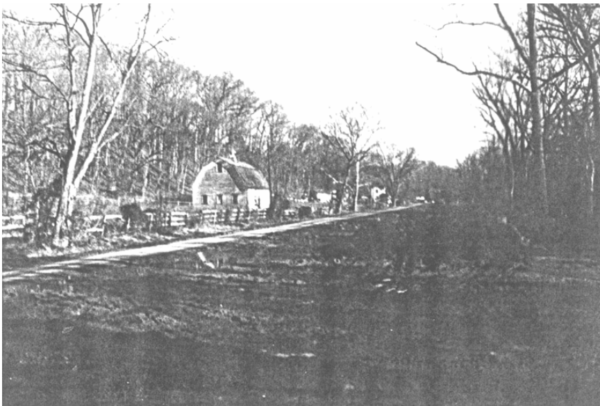
West end of project area in 1974 with view of the barn and other structures sited along Pennyfield Lock Road where it parallels the canal. (CHOH, Beasley appraisal)
