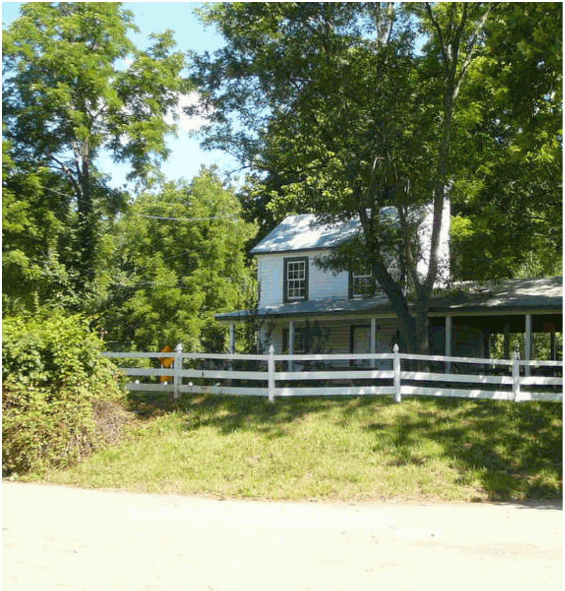
West House, south elevation. (CLP, 2010)
