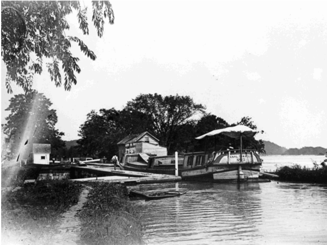
Lock 24 and Seneca Aqueduct looking east. Note feed store and shed on the river side. (circa early 20th century, CHOH Photo Files)
