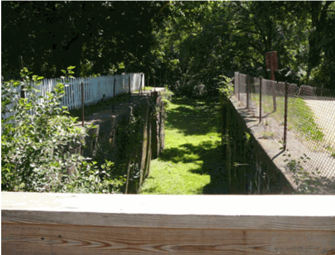
Lock 24, looking east. (CLP, 2010)
