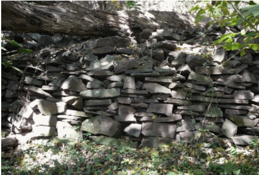
Loading and Retaining Walls at Mile 23.65. (NPS/LCS 2006)
