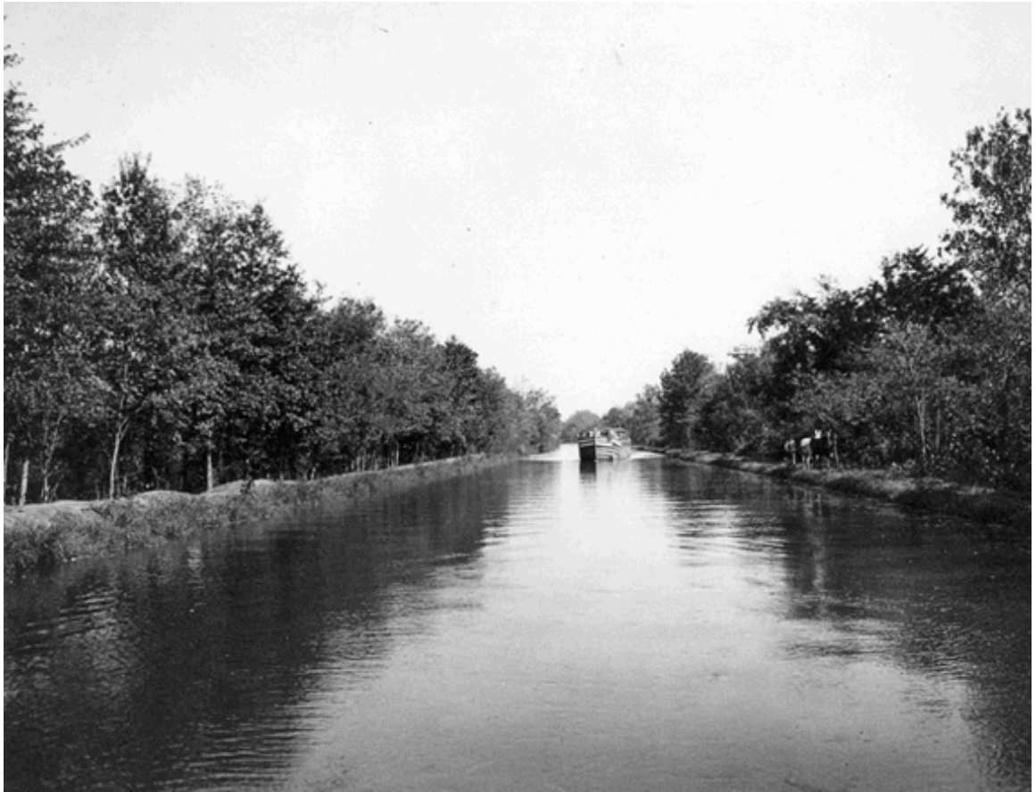
Canal in the vicinity of Seneca Lock, looking east. (Circa early 20th century, CHOH Photo Files)
