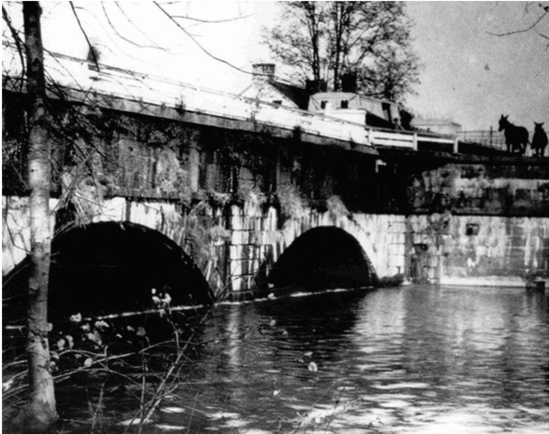
Seneca Aqueduct looking northwest. Note the iron fence and wooden fence along the river side. (circa early 20th century, CHOH Photo Files)
