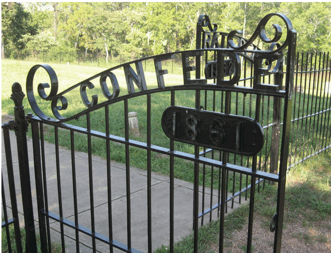
Gate detail (NCR CLP 2009) (Fig. 18)
