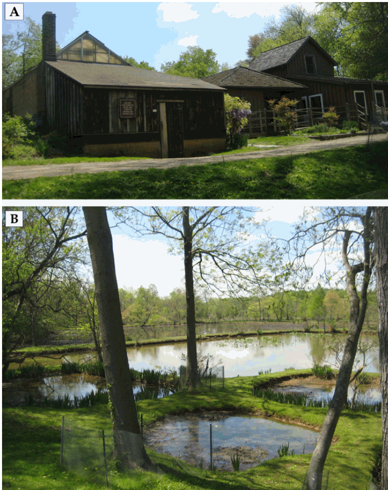
Figure 25. (a) Looking east at Hothouses 1 and 2 and the Administration Building; (b) Looking southwest across the ponds, with tree fencing in foreground (NCR CLP 2010). Note silting in foreground, and erosion on the far edge of Pond 4.
