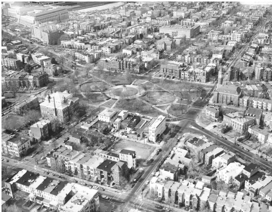
Aerial view of Stanton Park. National Park Service photograph by Jack E. Boucher, HABS, 1993.
