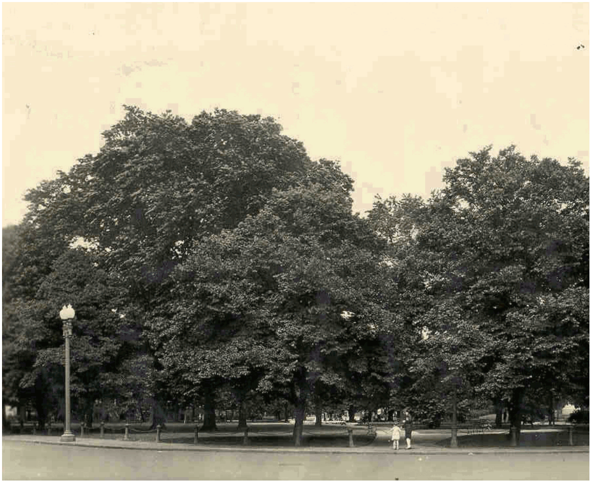
Perimeter view of Stanton Park. Note twin-twenty Washington Standard lights and standard Office of Public Buildings and Grounds bollards surrounding the park, 1927. (NCR, Division of Lands, Resources and Planning, Reservation File 15.)
