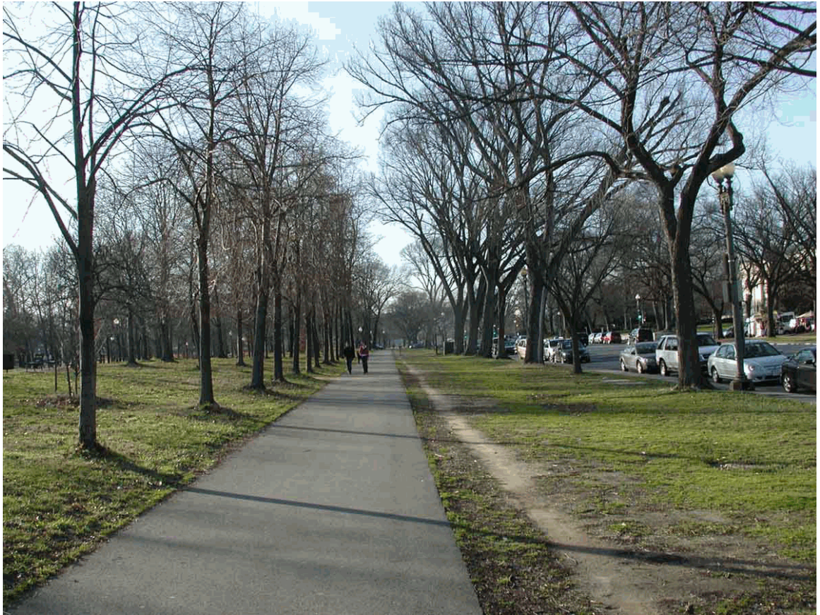
This wide asphalt sidewalk along Constitution Avenue replaced the former Tourmobile drive. A jogging trail has been worn into the ground beside it. A narrower sidewalk along the curb is barely visible in this photo. (Jan. 2007; CLP file)
