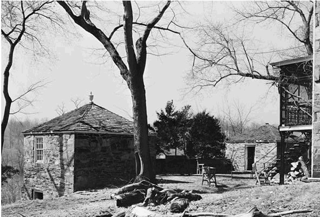
The two stone outbuildings and the south side of the house created a utilitarian outdoor service area. From circa 1935 Historic American Buildings Survey photograph.
