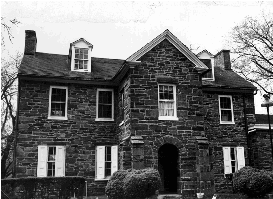
This photograph of the northern façade of the house was taken after the 1936 rehabilitation. Characteristics typical of the Colonial Revival style include the shutters and foundation plantings.
