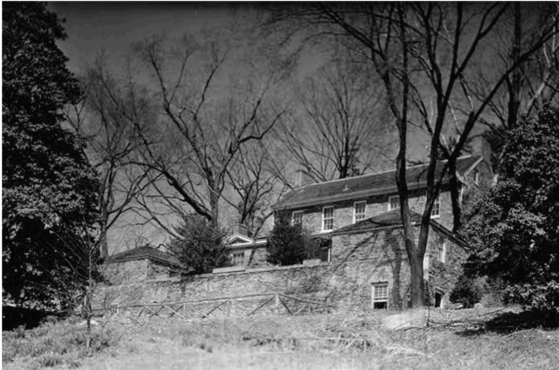
Circa 1935 Historic American Buildings Survey photograph of retaining wall formerly serving as rear wall of greenhouse, which had been removed by this time.
