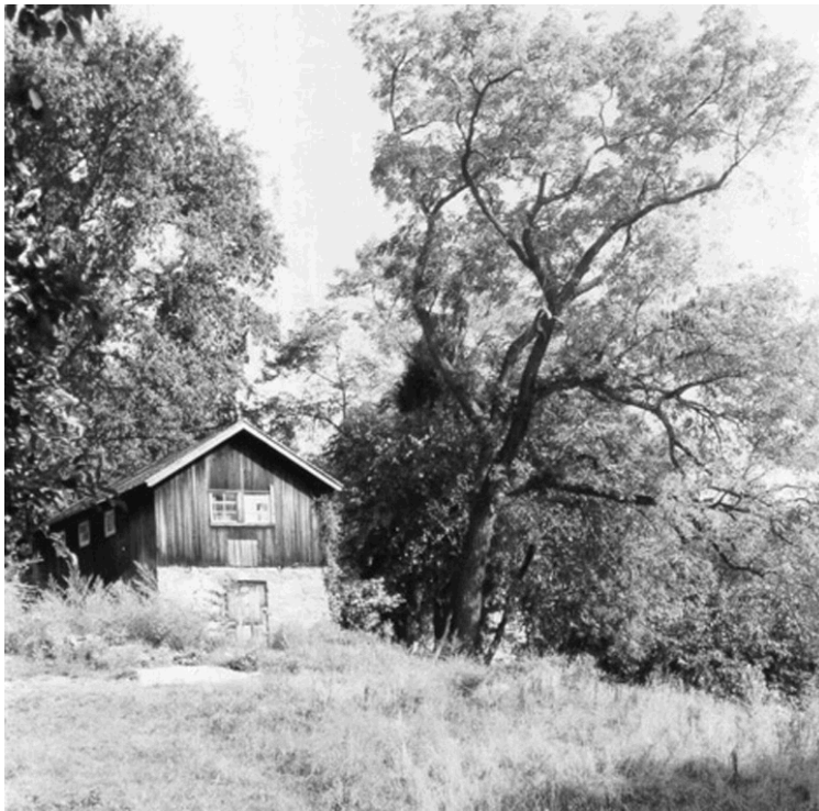
This 1993 view to the west side of the carriage house/stable includes examples of mature vegetation on the site.
