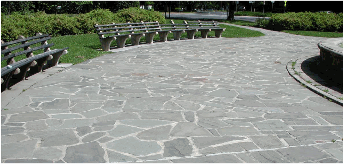
Repaired flagstone plaza eliminated severe cracking (CLP digital photofile, May 26, 2005).
